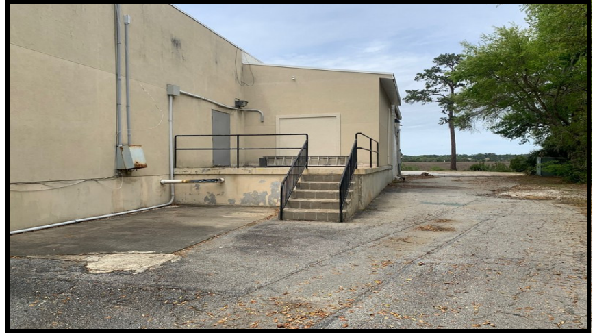
Westerly Oriented View Along The Northern (Rear) Building Elevation
