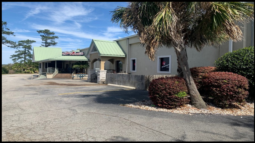
Northerly Oriented View Along The Western Building Elevation
