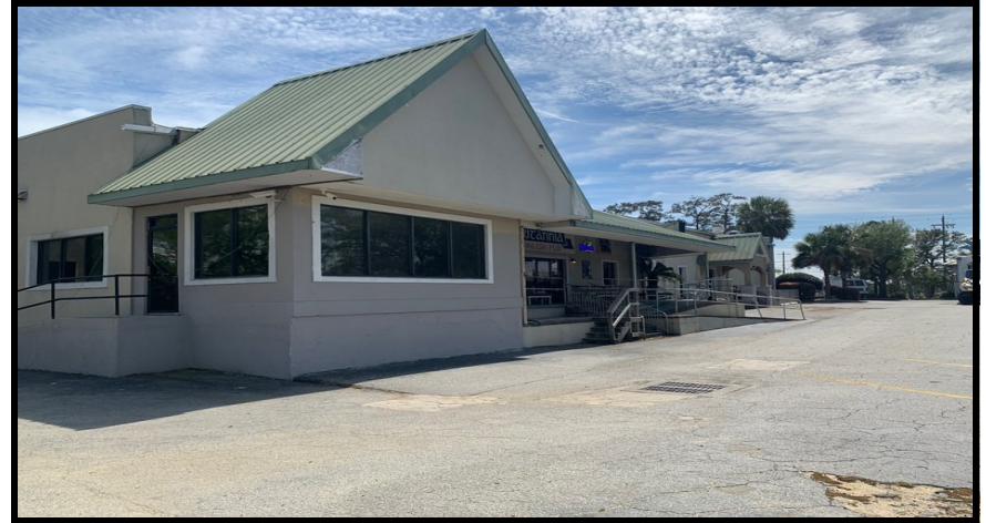
Southern Oriented View Along The Western Building Elevation
