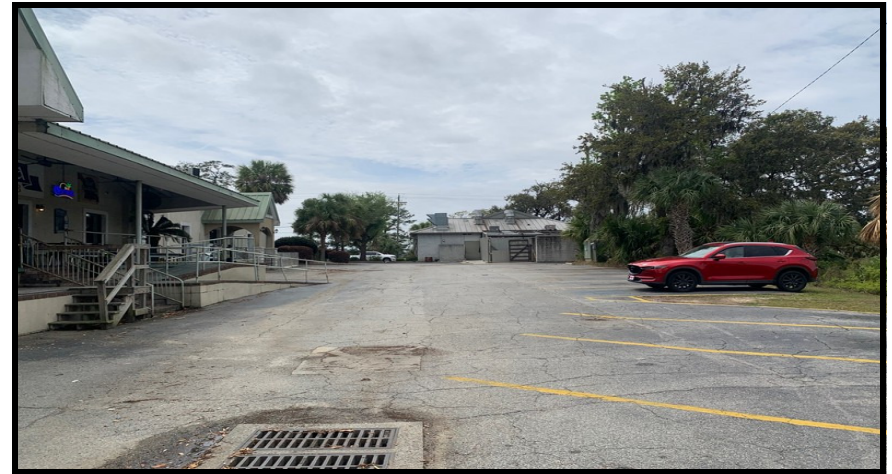
Northerly Oriented View Along An Internal Drive Along The Building Western Elevation
