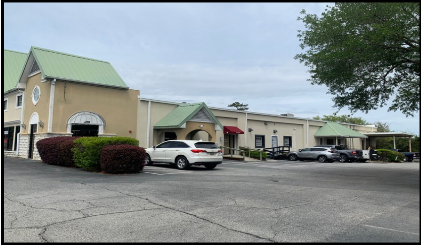
Northwesterly Oriented View Along The Eastern Building Elevation
