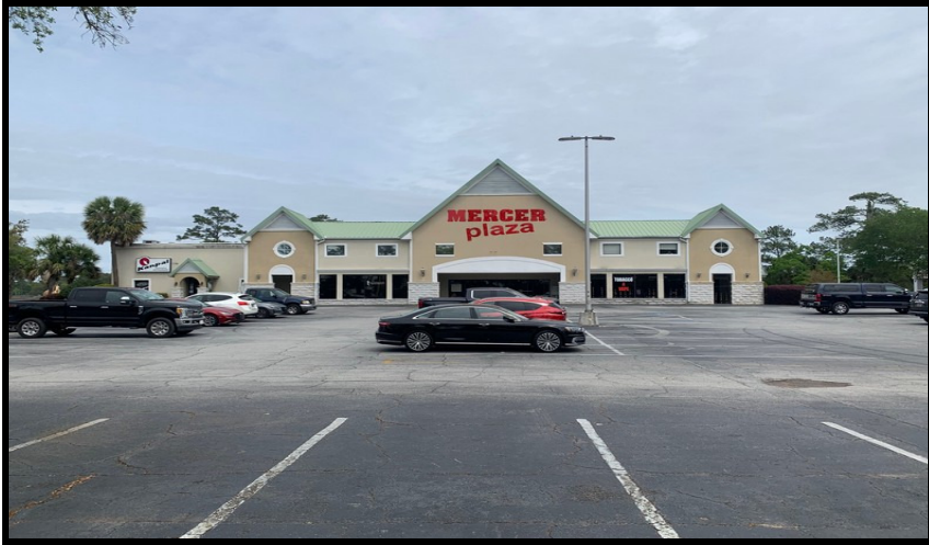
Northerly Oriented View Of The Southern (Front) Building Elevation
