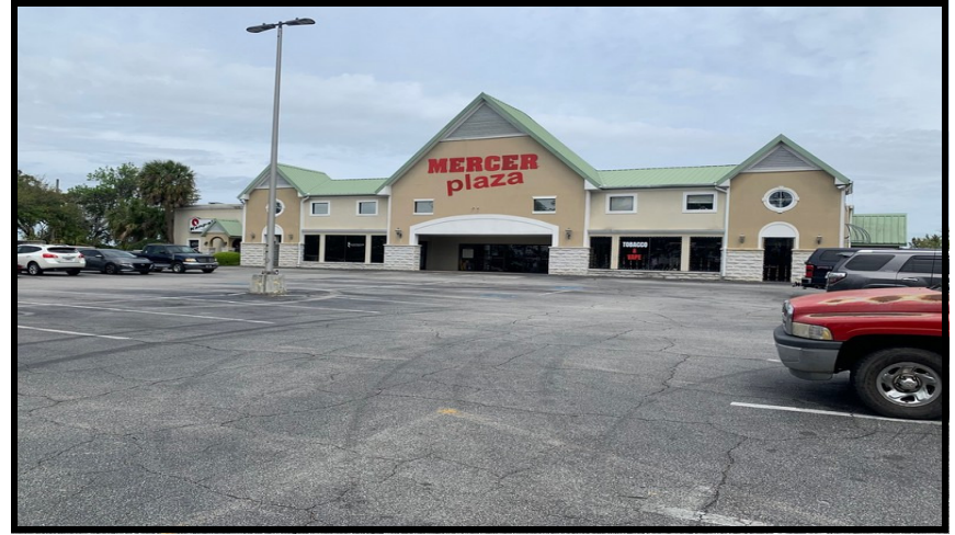
Northwesterly Skewed View Of The Southern (Front) Building Elevation
