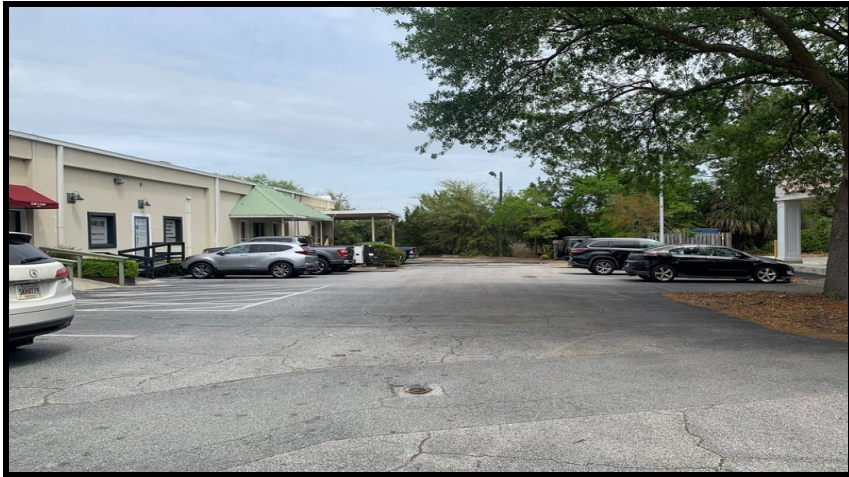
Southerly Oriented View Of An Internal Drive Along The Building Eastern Elevation
