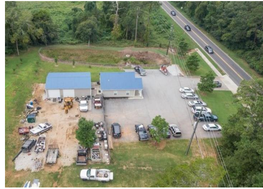
Improved acre, oversized stormwater detention
