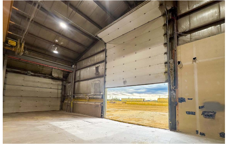
5 Oversize Grade Loading Doors
