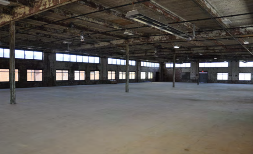
Building 4 - Main Level
