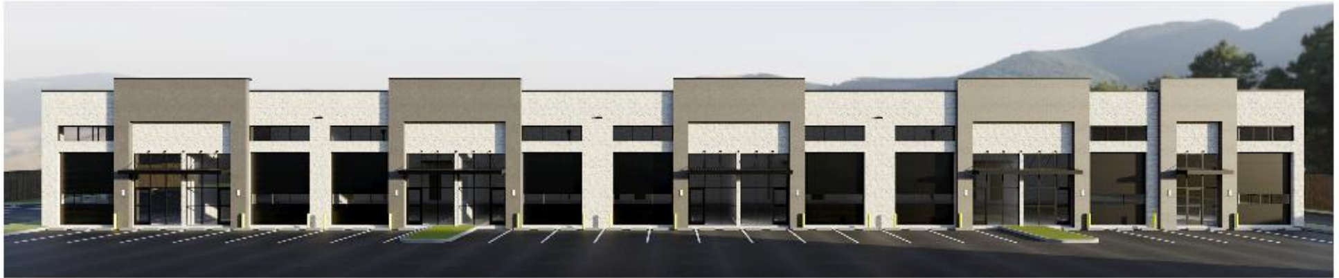
FLEX BUILDING FRONT VIEW
