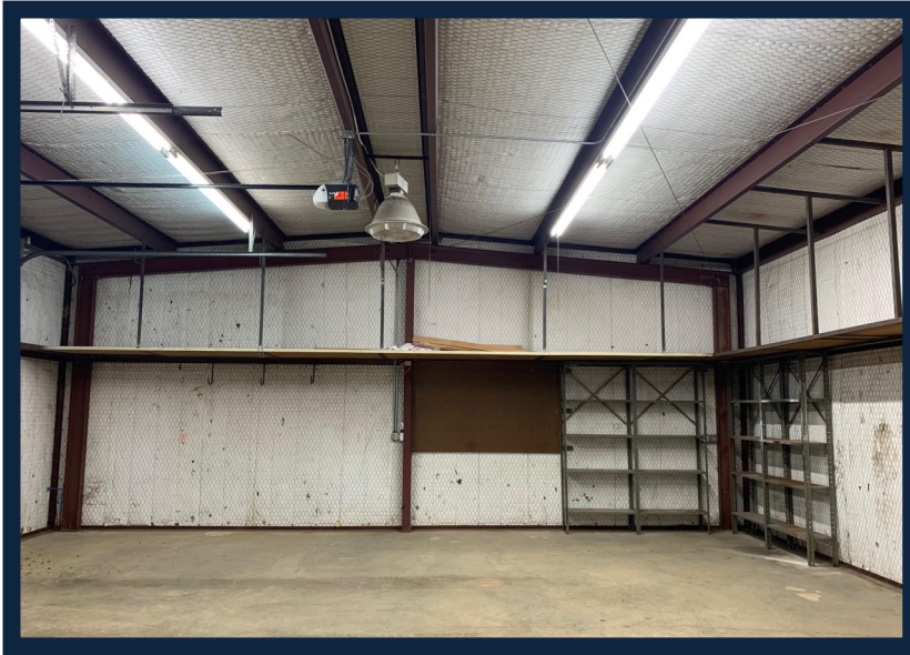
Rear of Warehouse with Ample Shelving
