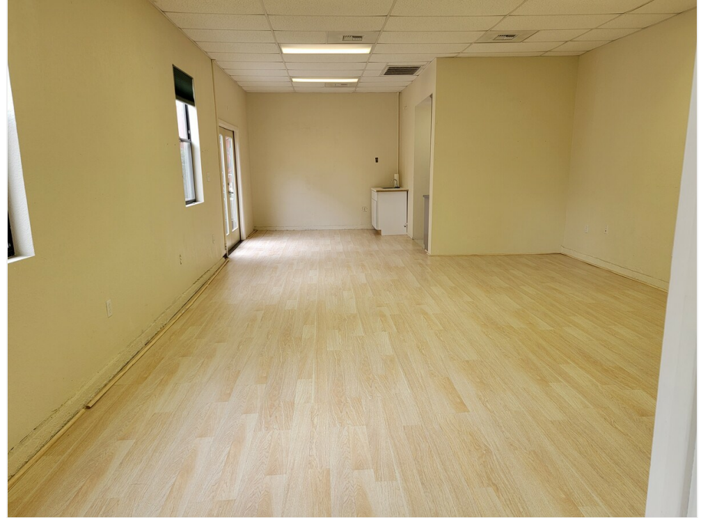
Back Room view to Restroom
