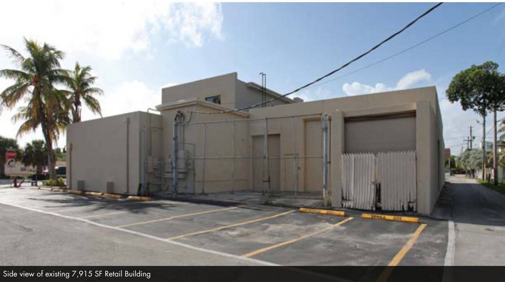
Existing 7,915 SF Retail Building
