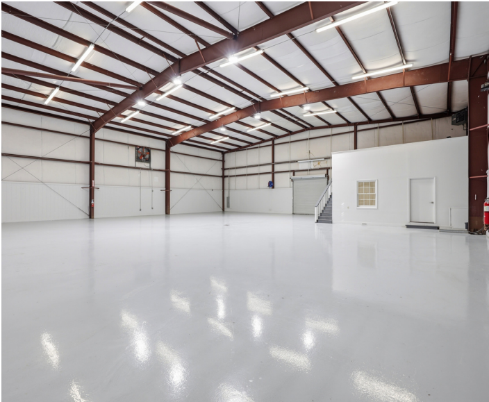
MAIN BAY · CLEAR-SPAN INTERIOR
