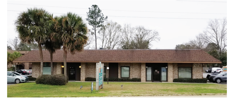
EXISTING BUILDING - 1 STORY FRONT VIEW
