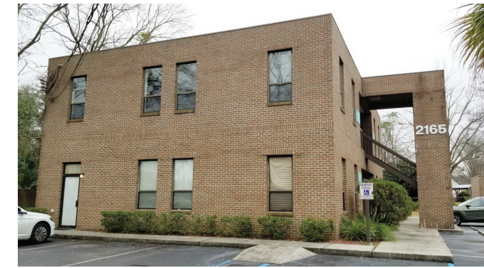
EXISTING BUILDING - 2 STORY SIDE VIEW
