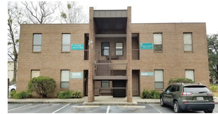
EXISTING BUILDING - 2 STORY FRONT VIEW
