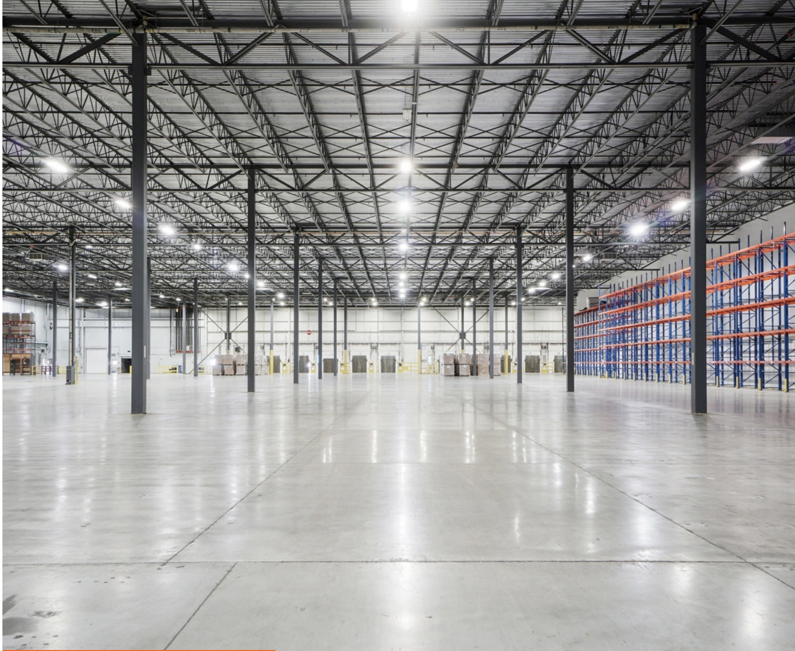
/±134 201 SF Industrial area
