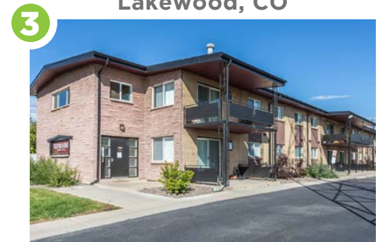
9885 W 21st Ave Lakewood, CO
