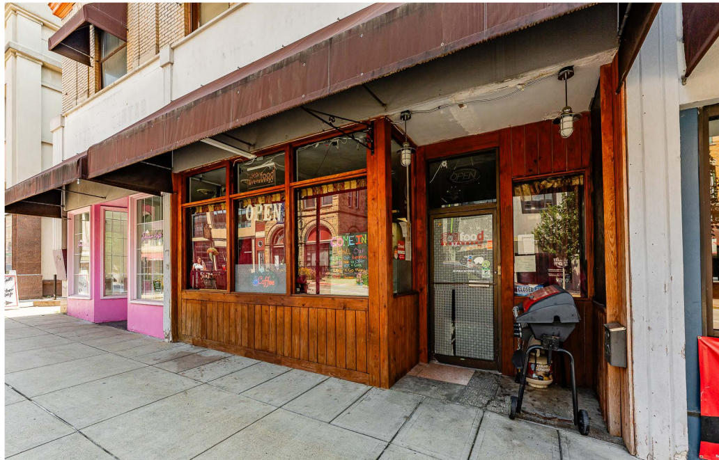
Front View of the Building from High Street.
