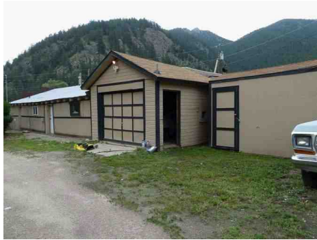
Front viewing southeast
