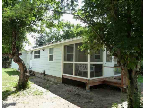
Front viewing southeast
