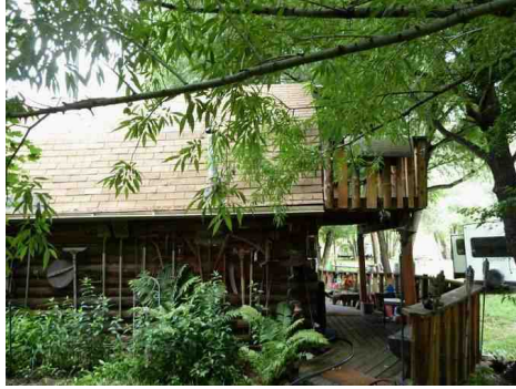
Front and south side
