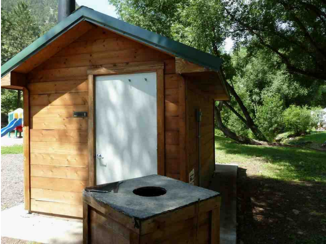
One of two restroom buildings
