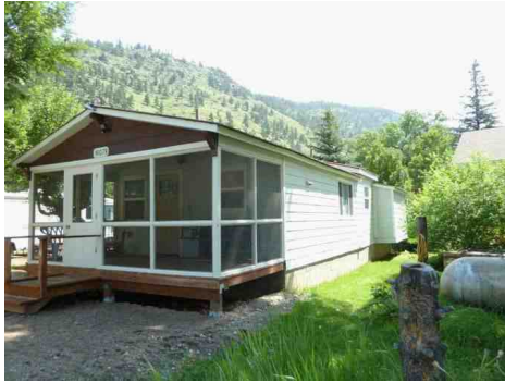
Front viewing northeast
