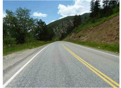
Viewing south along County Road 4
