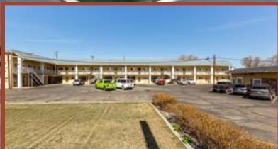
1349 IDAHO STREET SUBJECT PROPERTY
