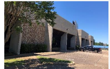
SUITES G-L Runs north-south with east-facing entry.
