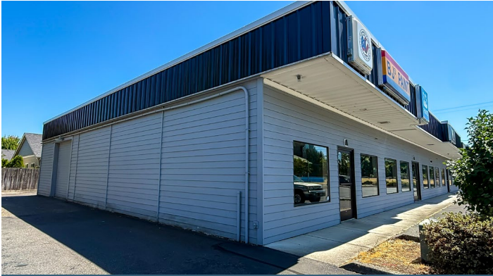
SUITE A - EXTERIOR WITH VIEW OF ROLL-UP DOOR
