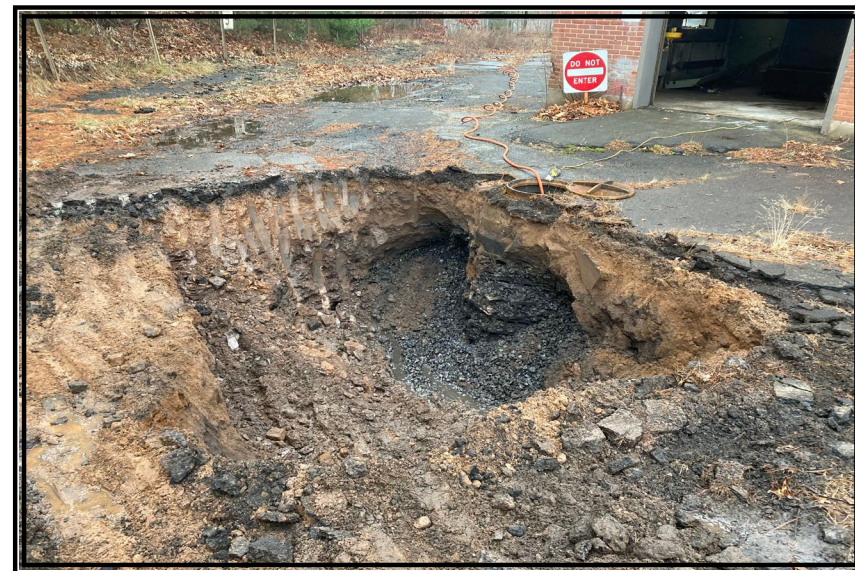
Photograph 6 Dry well at RA-6
