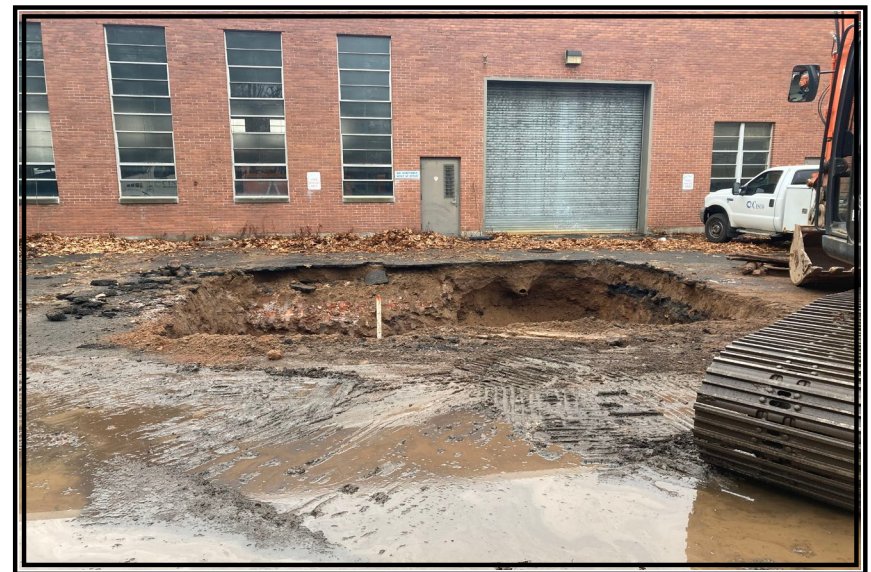
Photograph 4 Excavation at RA-5
