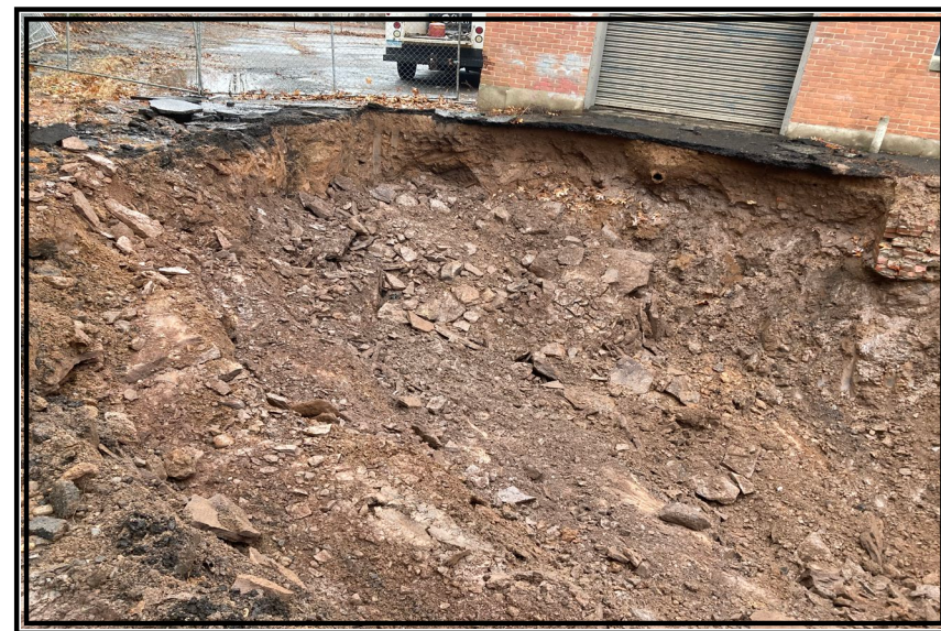
Photograph 8 Additional soil removal at RA-6
