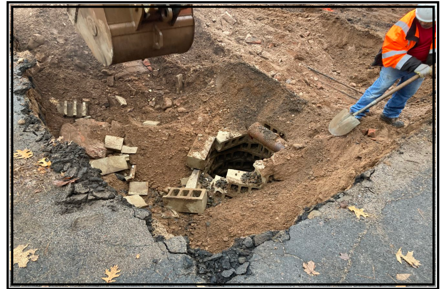
Photograph 2 Dry well at RA-5
