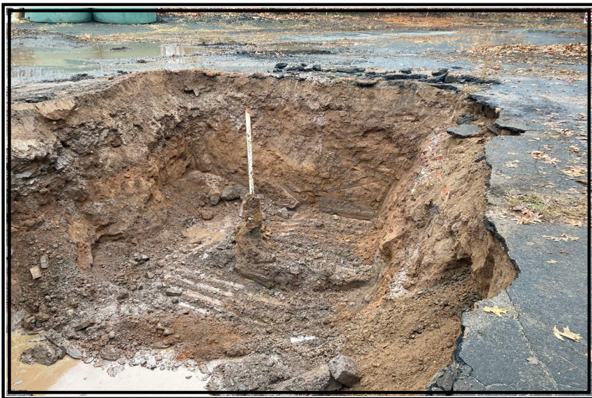
Photograph 3 Excavation of RA-5
