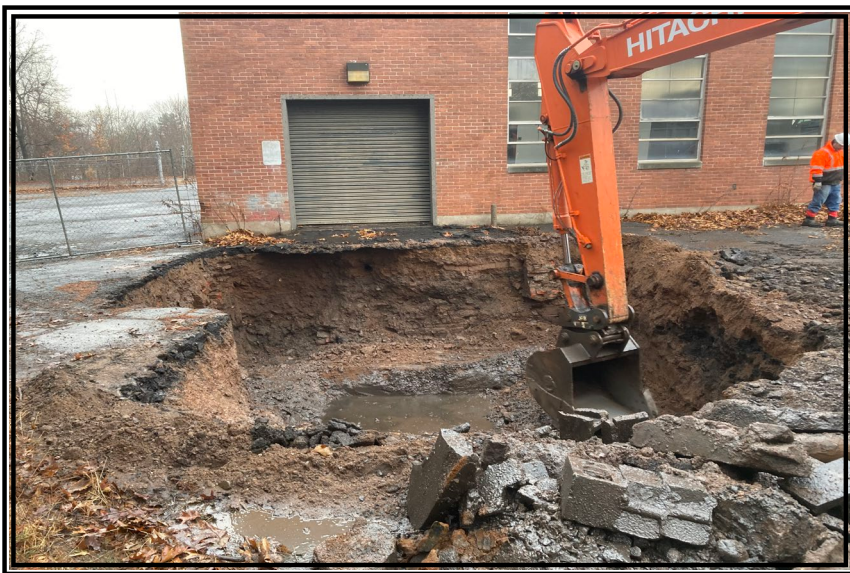
Photograph 7 Initial RA-6 excavation limits
