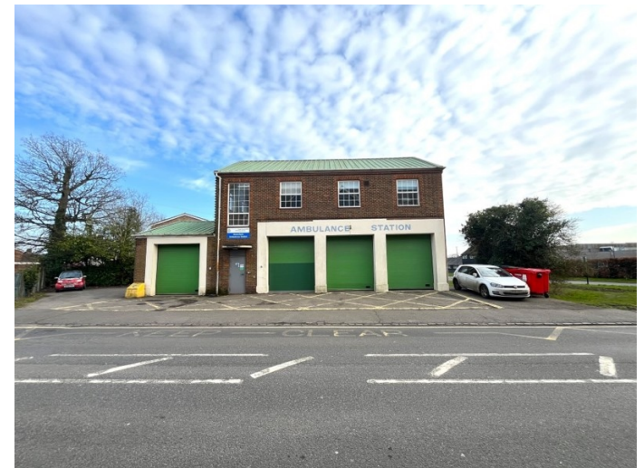
Front of Site with parking areas on left and right
