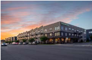
BEXLEY SILO BEND 193 apartments
