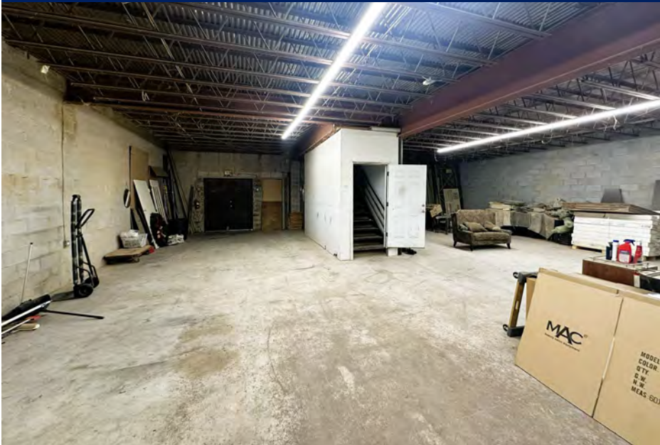
Bay 5 – Lower Level (Vacant at Closing)
