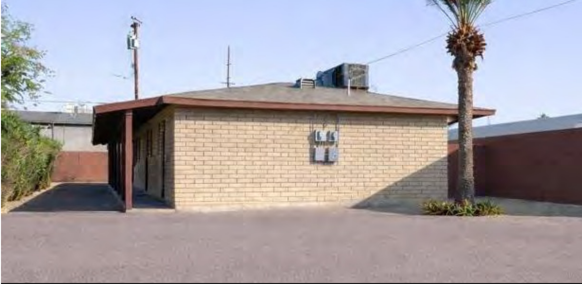
SLUMP-BLOCK EXTERIOR AND PARKING AREA
