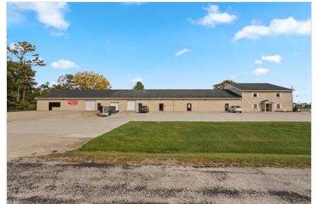
Front of Structure
