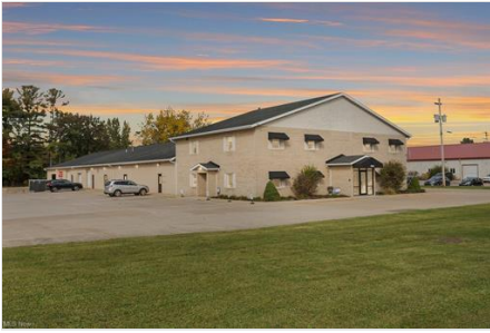
Front of Structure
