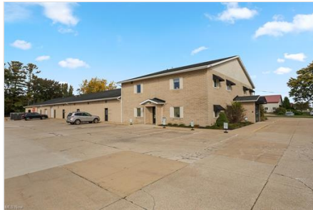
Front of Structure
