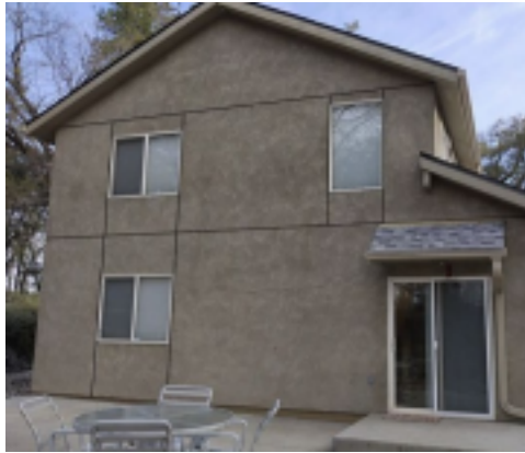
Figure 2: Stucco and EIFS control joints are prohibited
