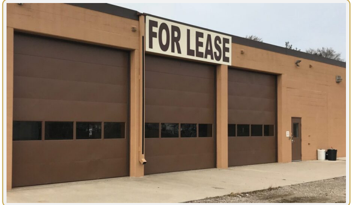
Building Exterior — Bay Doors & Frontage
