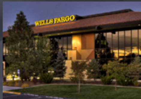
5340 Kietzke Lane, Reno 55,917 SF Class A Office
