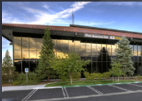
5310 Kietzke Lane, Reno 55,387 SF Class A Office
