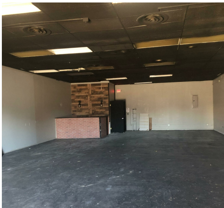
341-343 Hastings: 3,000 square feet
