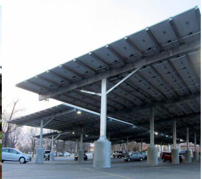
Solar Panel Covered Parking
