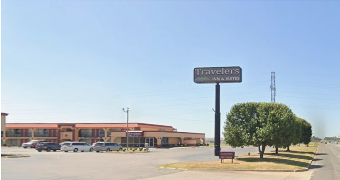
Front elevation and monument signage, S. MacArthur Blvd.
