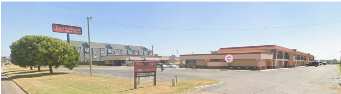
Site overview showing building footprint and parking. Source: Google Street View, 2026.
