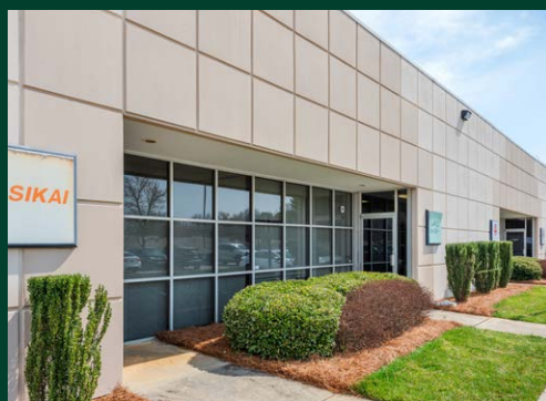
PRECAST CONCRETE AND GLASS FACADE
