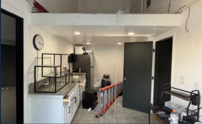
Rear plumbing connectivity & kitchenette area
