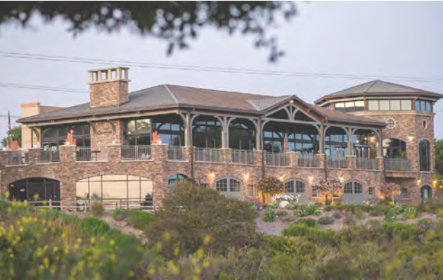
AVARIA The Crossings at Carlsbad
