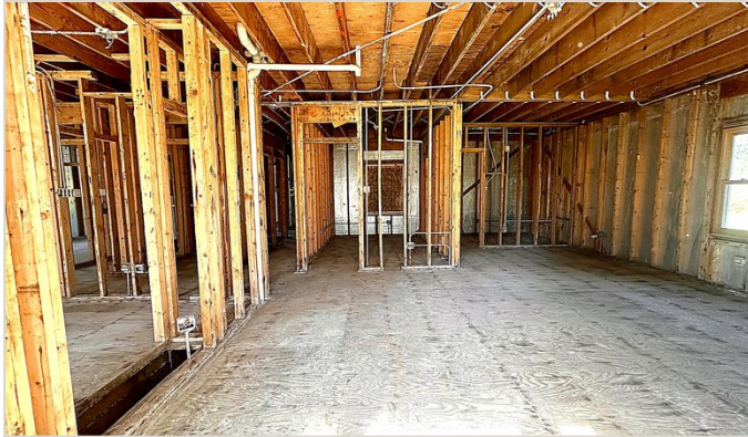
Open Floor Plan Main level, framed and ready for build-out
