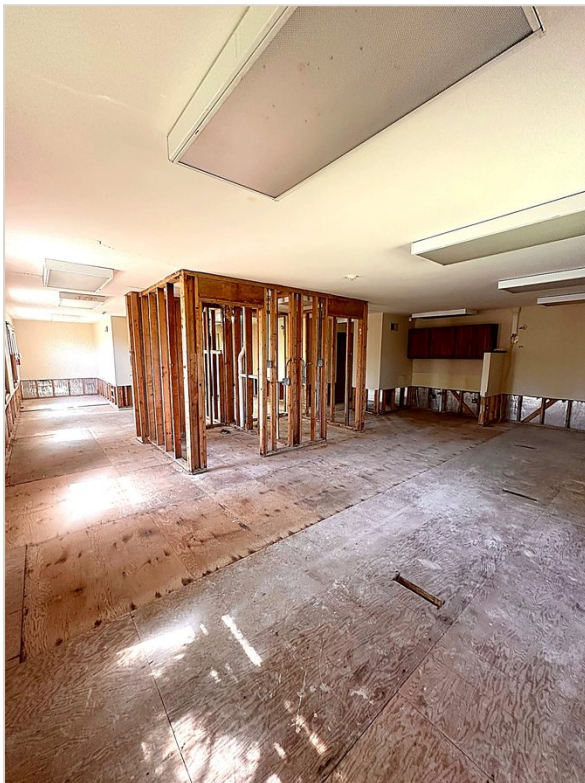
Interior Framing Detail Structural framing and rough mechanicals
