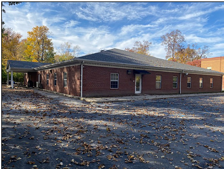
Former drive thru
