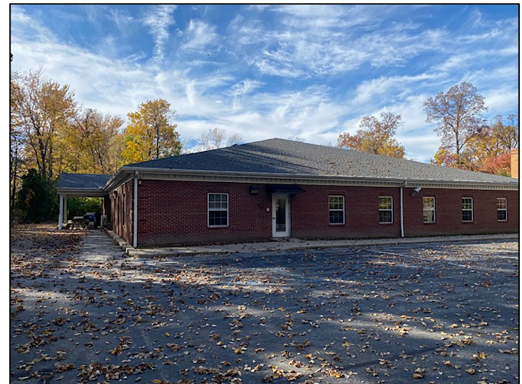
Rear section entry
