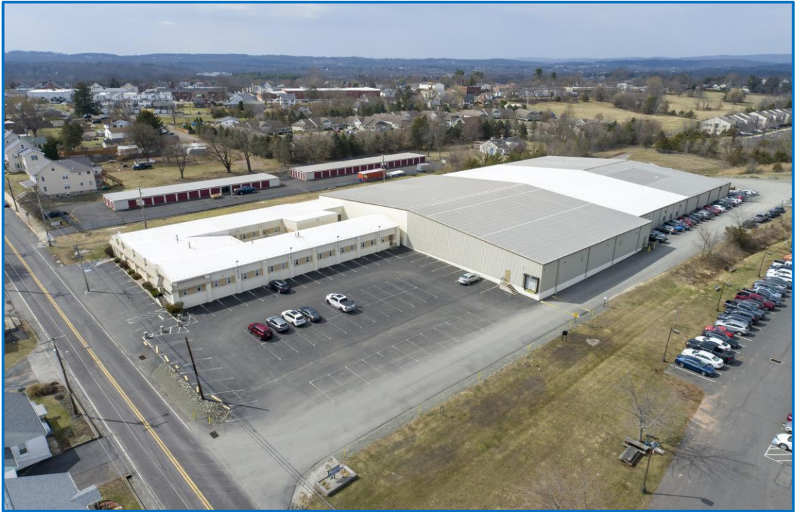
BUILDING FRONT VIEW:
