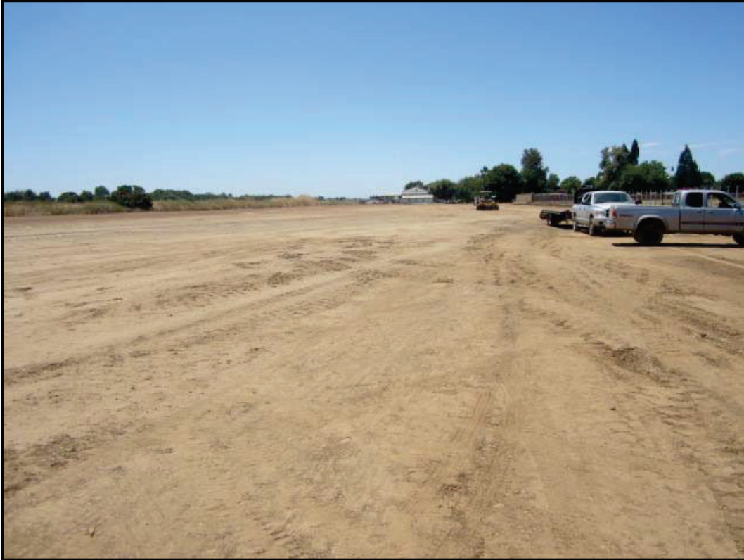
Lot #17 View Looking Southwest
