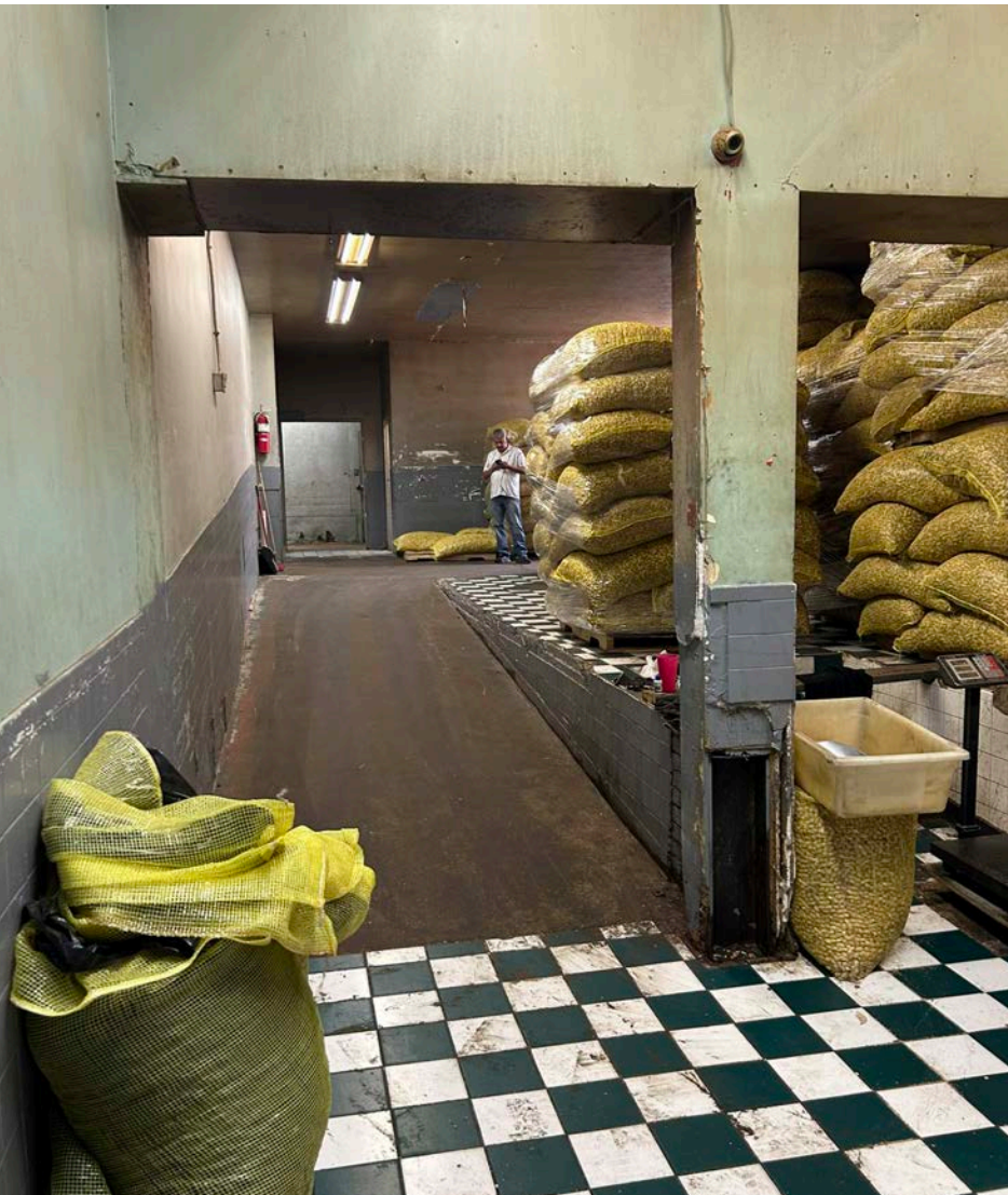
Buyer to verify all infrastructure, permit status, and equipment condition during due diligence. Refrigeration compressors in Unit A are currently non-operational and should be assumed to require replacement.
