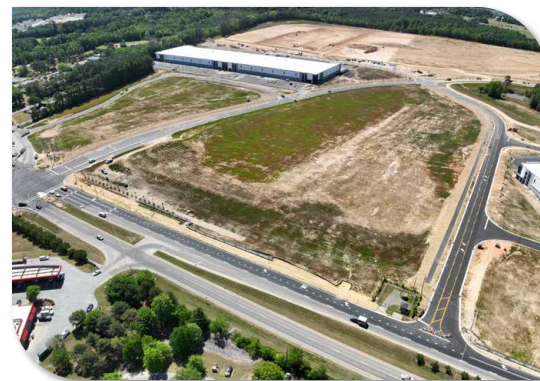
CONSTRUCTION PROGRESS AS OF APRIL 21, 2026
