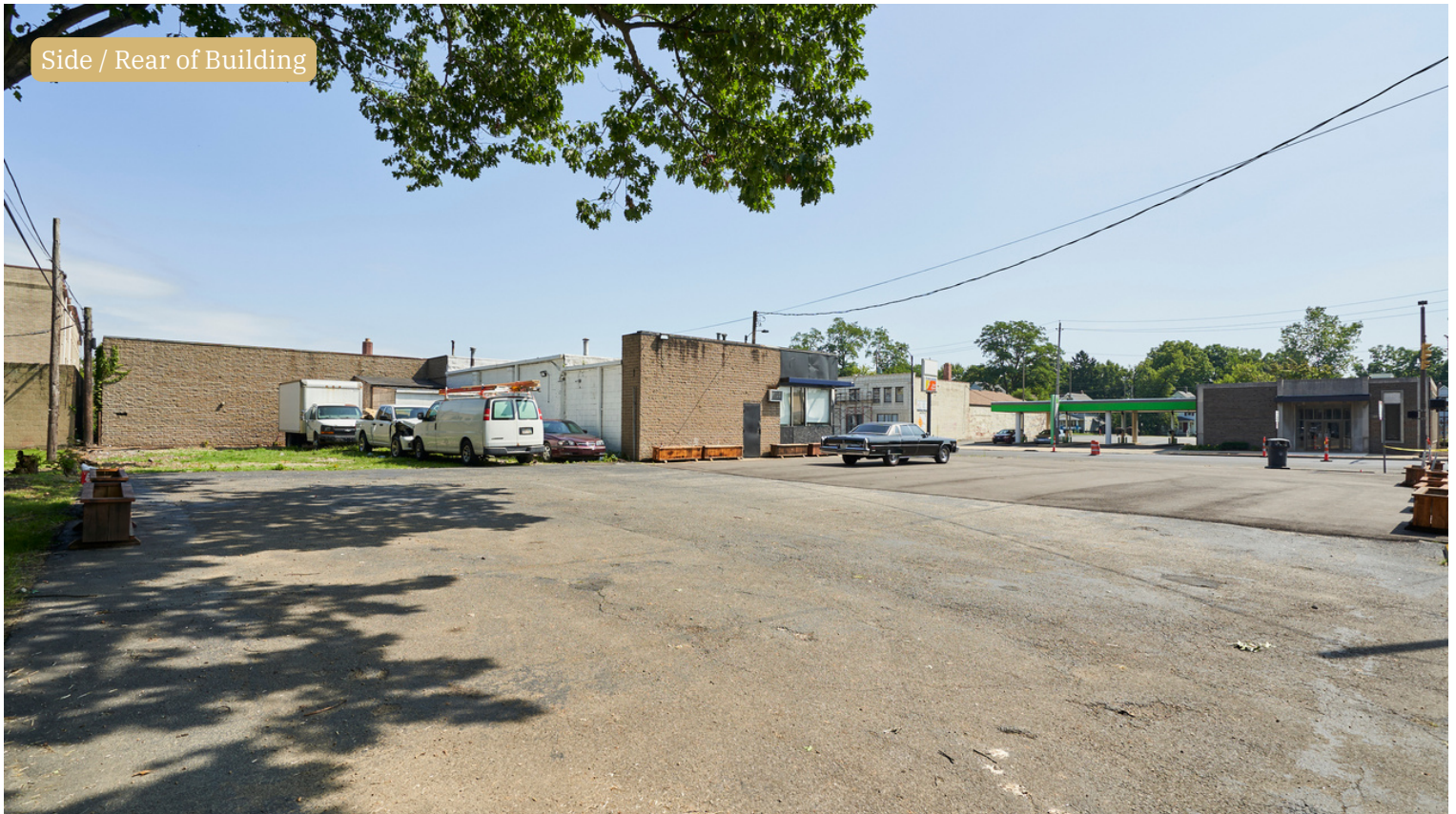
Front Building /Side of Building
