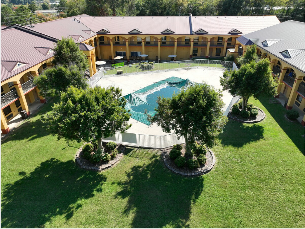
Aerial from Back of Property
