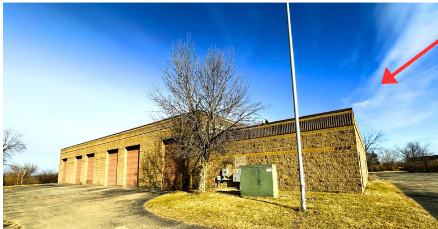
Former E-Check Facility
