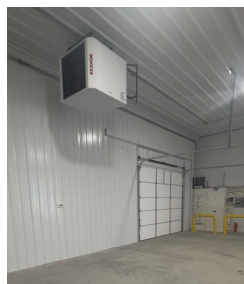
New floors & heaters
