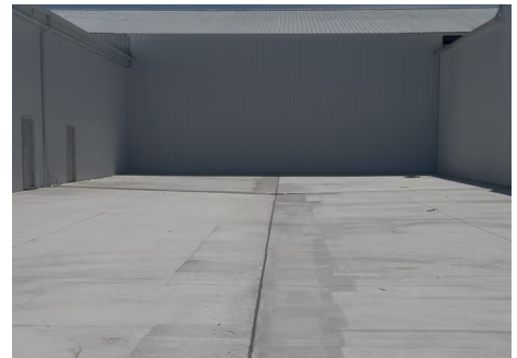
New concrete throughout the site
