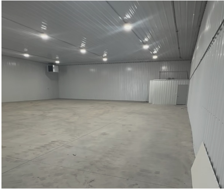
Remodeled interior – new floors, insulation & lighting
