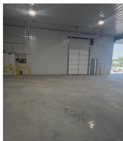
Drive-in & dock loading
