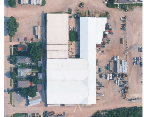
Aerial – 804 Grant Ave complex & yard
