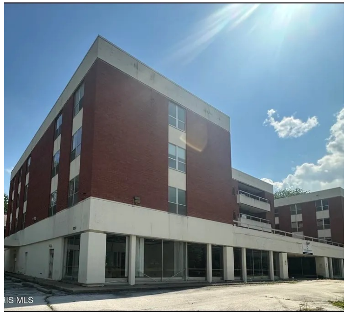
Side elevation / storefront-level facade
