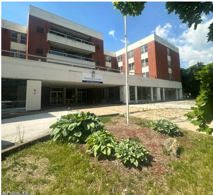
Collingwood frontage / principal entrance
