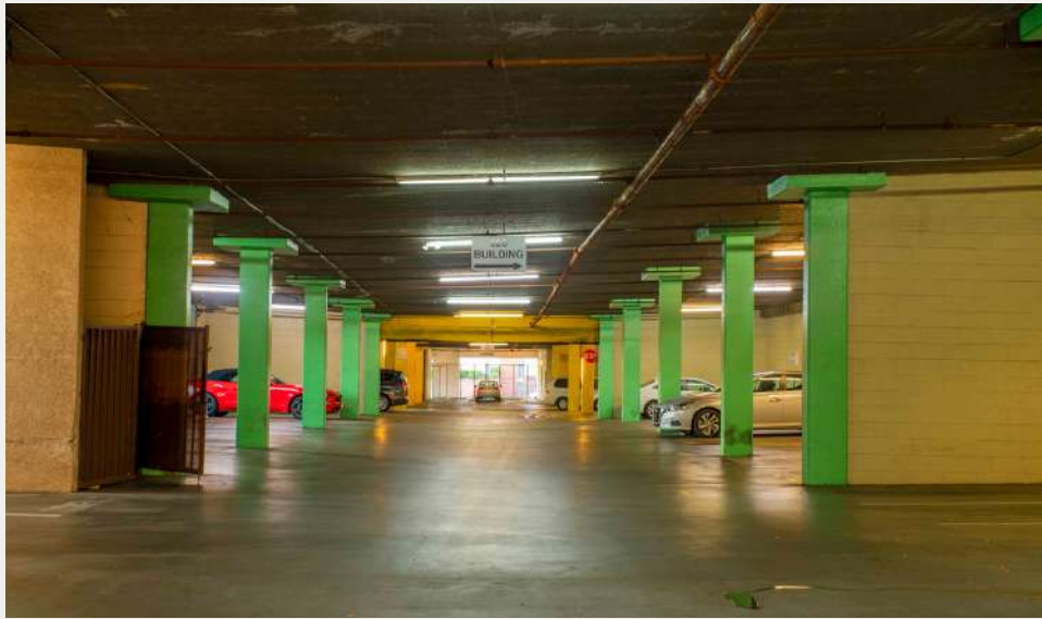
COMMONWEALTH PARKING ENTRANCE
