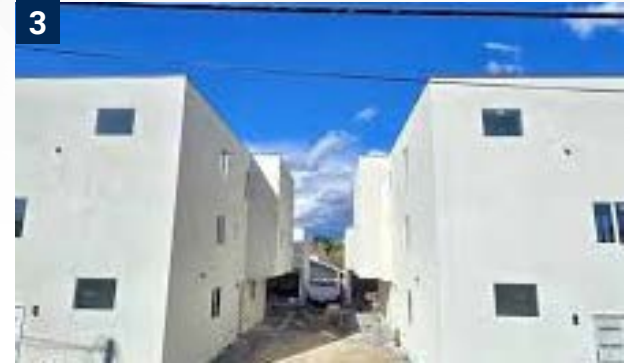
2415-2419 E 3rd Street Los Angeles, CA
