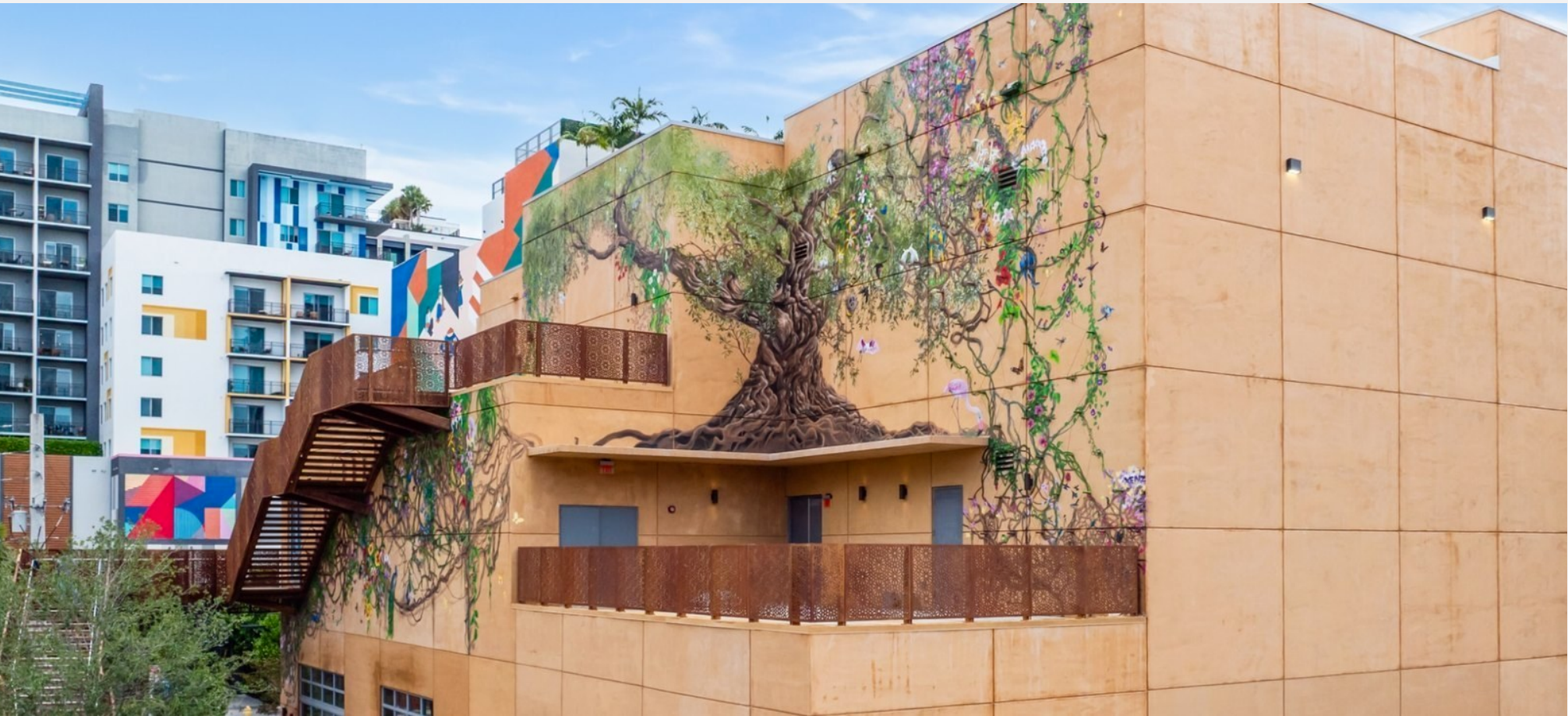
THE BANYAN — EAST ELEVATION, PAINTED FLOOR TO PARAPET
