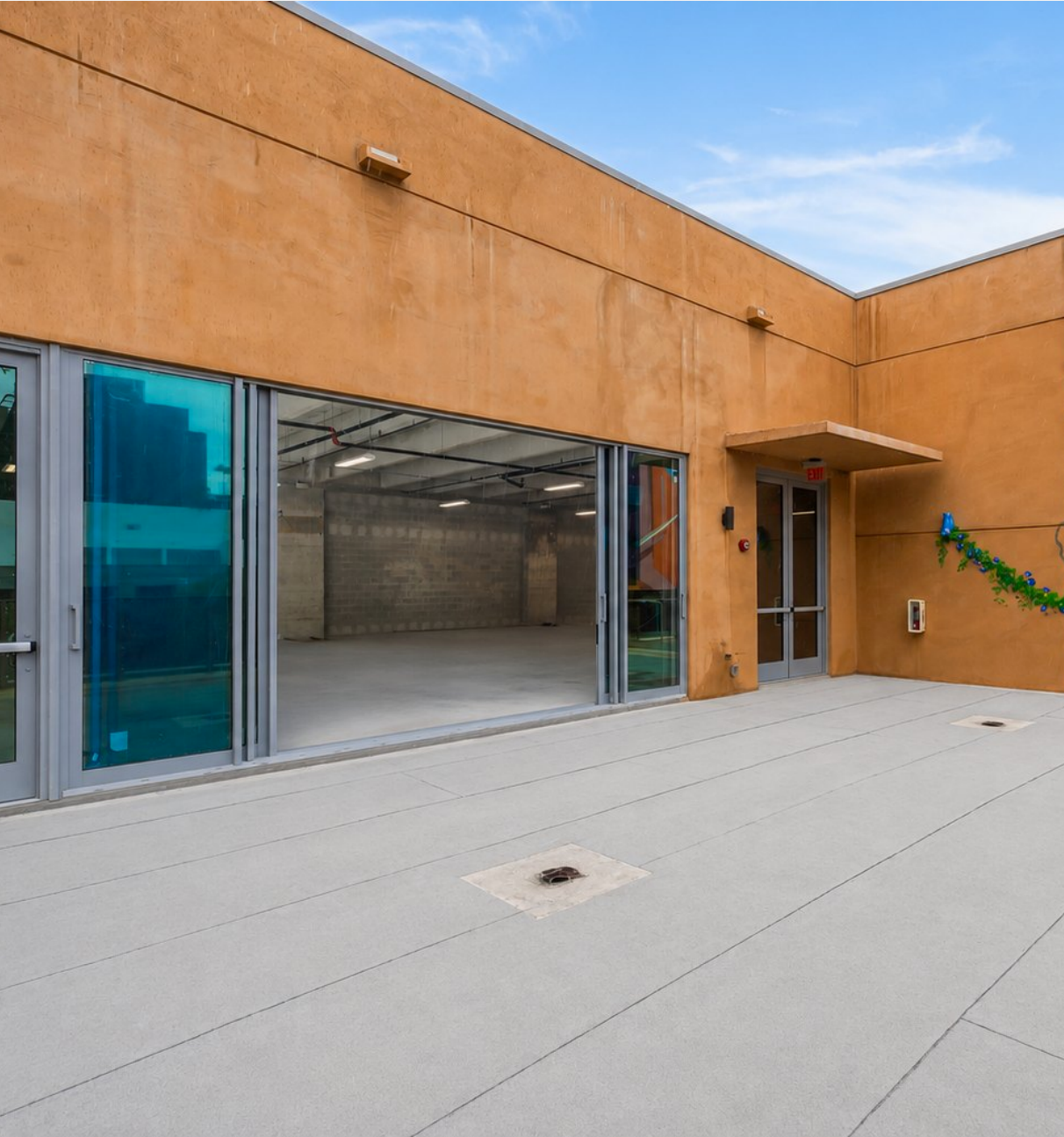
THE PRIVATE TERRACE — SLIDING GLASS WALLS OPEN THE FLOOR TO IT
