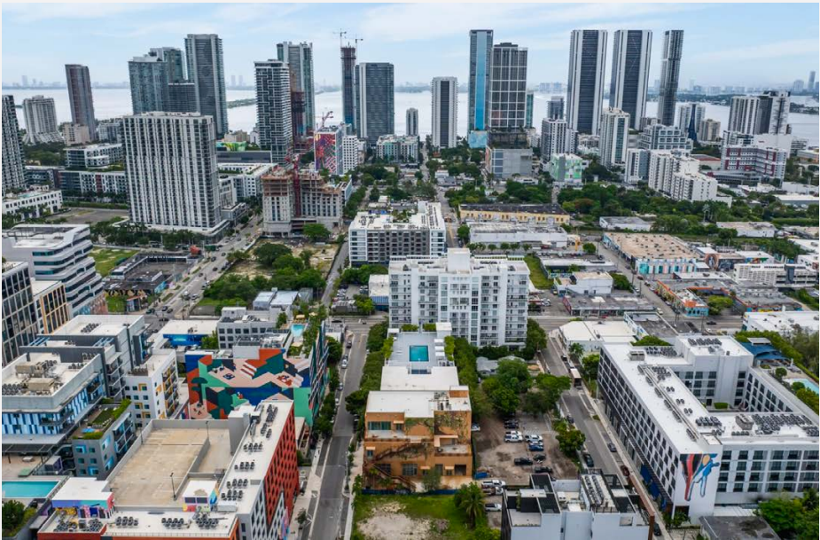
EAST — EDGEWATER TOWERS & BISCAYNE BAY
