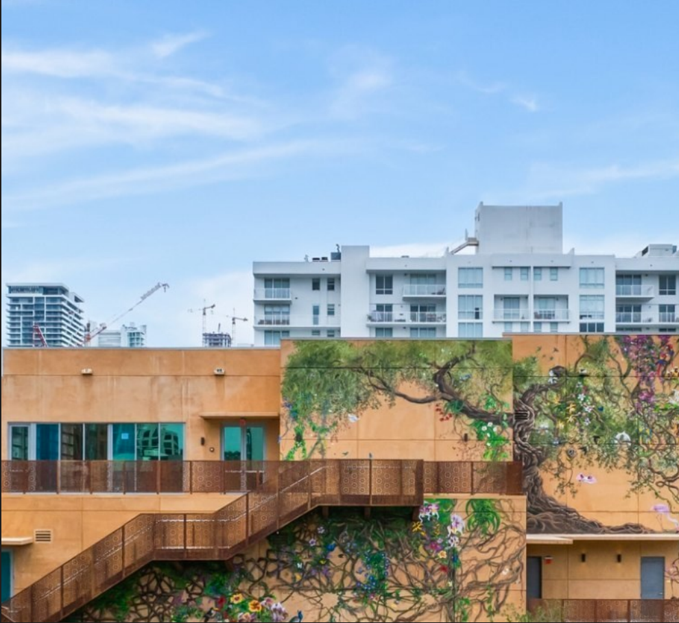
06 THREE STOREYS ON NW 28TH STREET
