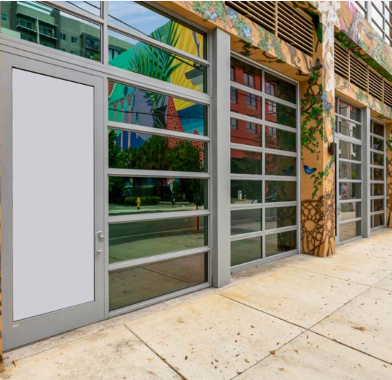
FLOOR-TO-CEILING GLASS AT THE SIDEWALK — THE WHOLE BAY READS FROM THE STREET
