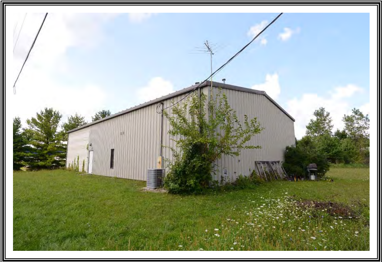
Northeast view of subject
