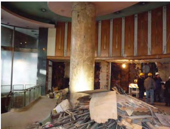
Image 33: First floor tenant space, view southeast.
