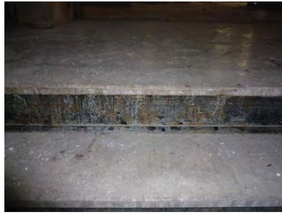
Image 68: Main stair, typical riser condition, floors 2 and above.
