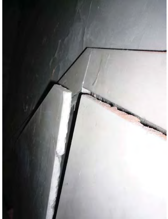
Image 72: Main stair, marble wainscoting 5 th floor (atypical).
