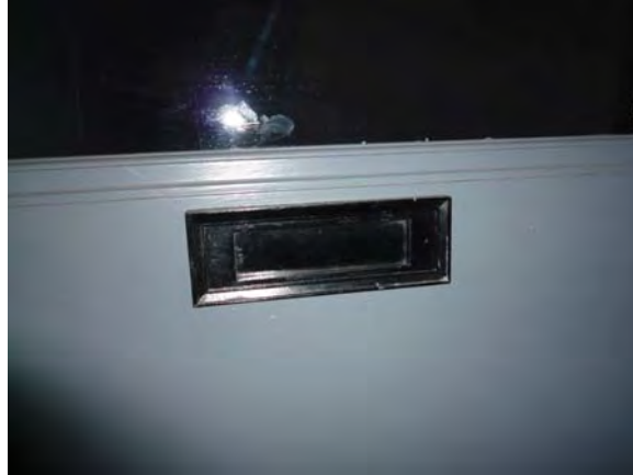
Image 88: Original mail slot, typical of office doors along main corridor.
