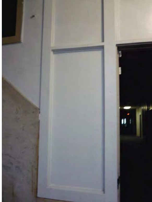
Image 66: Covered storefront, typical of west stair floors 2 through 21.
