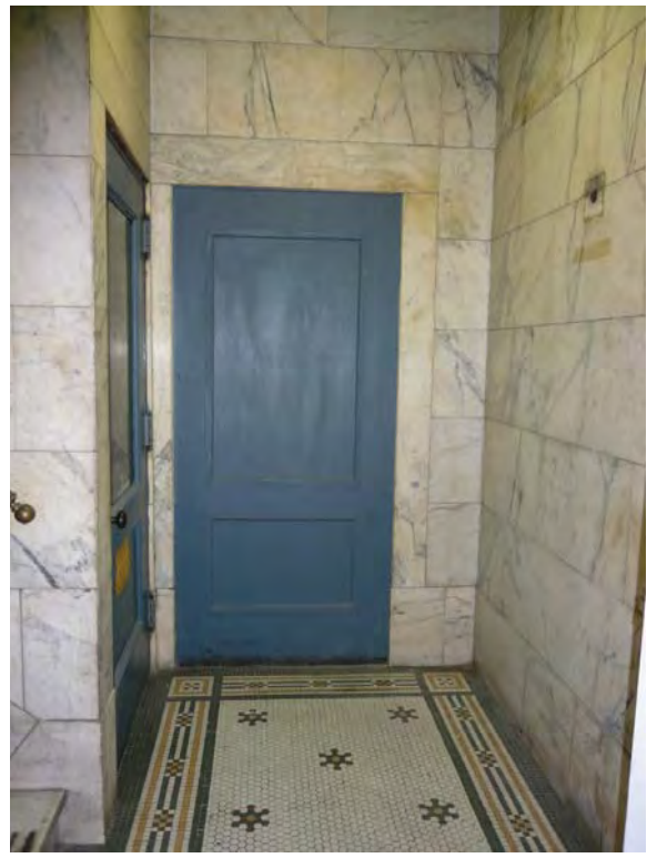
Image 62: East stair, original mosaic tile on first basement landing.
