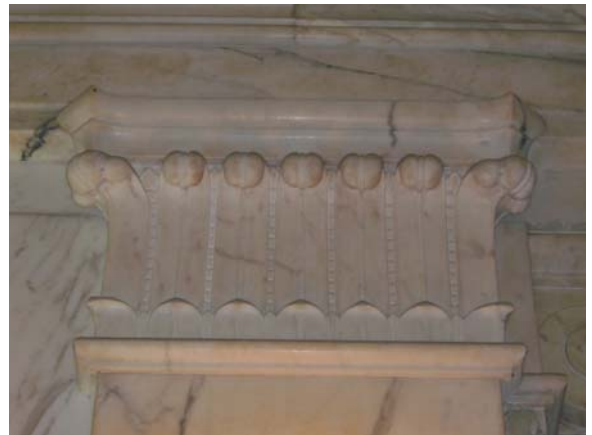
Image 44: Typical column capital, main lobby.
