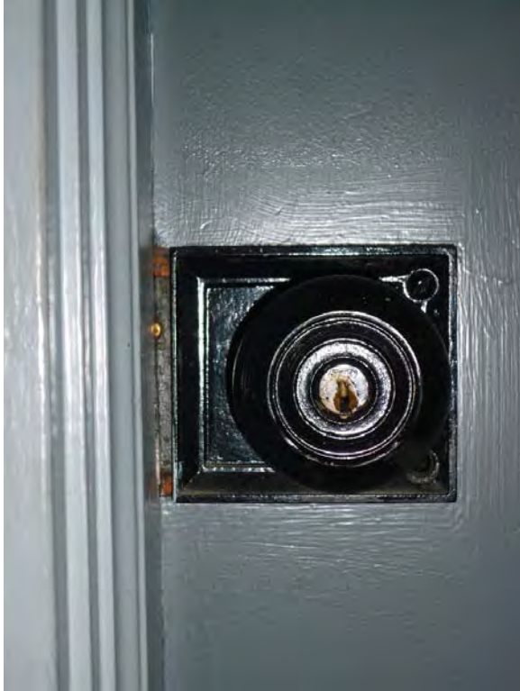
Image 87: Typical original door hardware.
