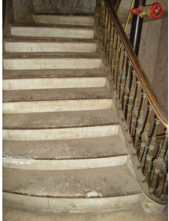
Image 80: Main stairway between basement and mezzanine. Note standpipe at right.
