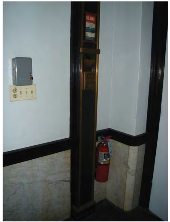
Image 86: Mail chute, east stair.
