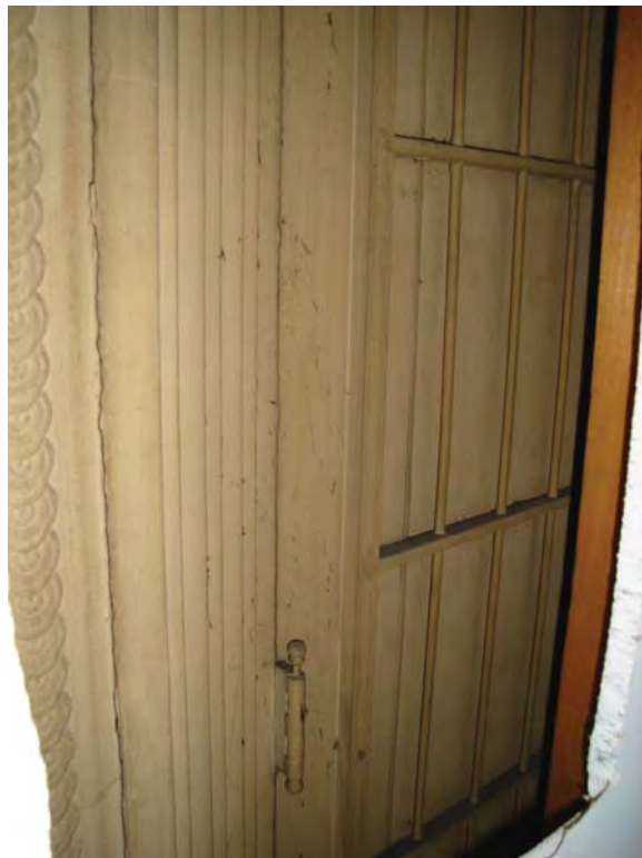
Image 50: 1 st basement, decoration remaining on elevator wall and doors.
