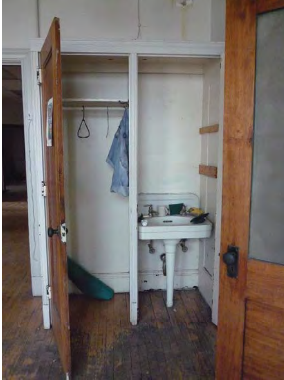
Image 75: 20 th floor, southeast office suite, water closet.
