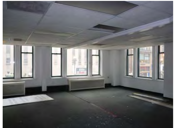
Image 94: Chicago windows, 2 nd floor. Typical of east and south façades, floors 2 through 4.
