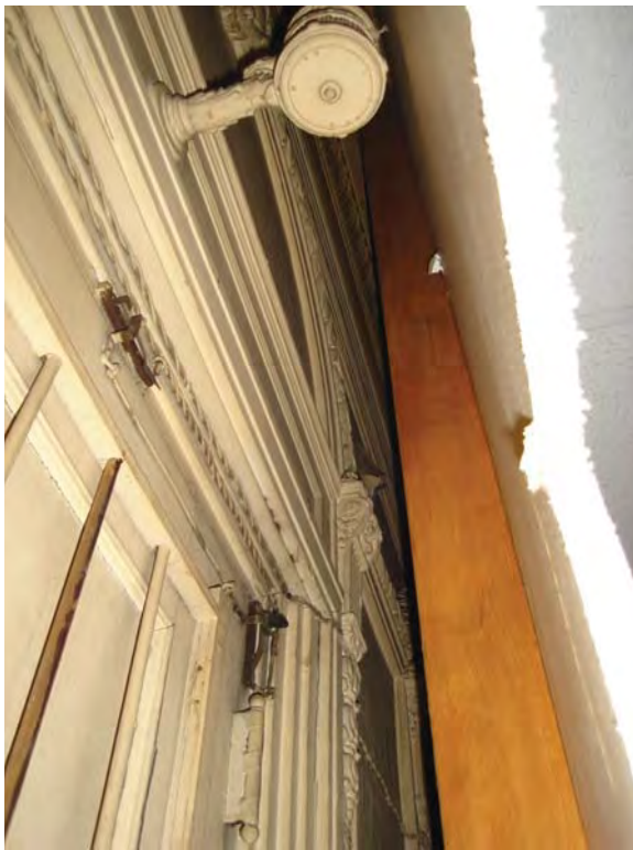
Image 49: 1 st basement, decoration remaining on elevator wall and doors.
