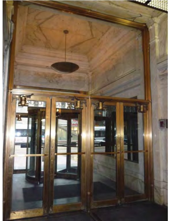
Image 36: Entry vestibule, view east from main lobby.
