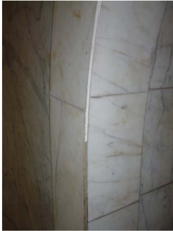
Image 104: Marble cladding, first floor lobby.
