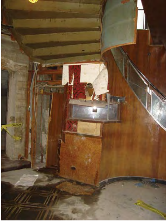
Image 75: Underside of decorative stair, first basement.
