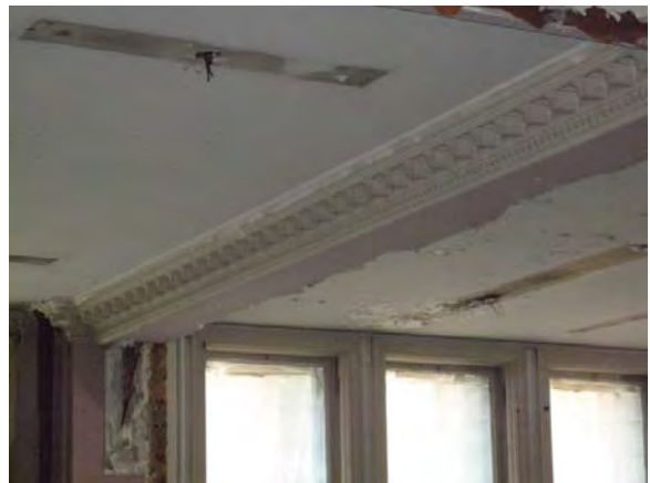
Image 50: Decorative ceiling beam, 8 th floor.
