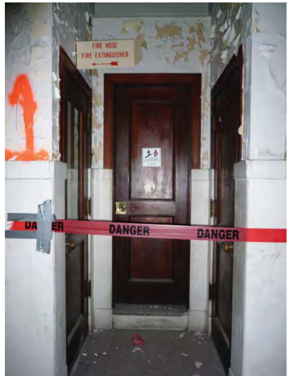
Image 58: 11 th floor utility closet doors. Typical of floors 2 through 15.
