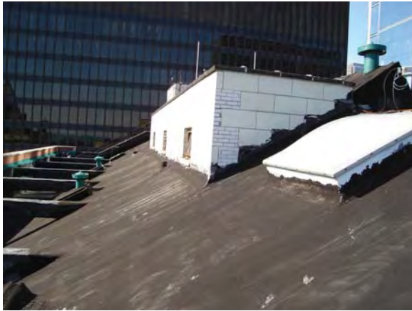
Image 99: Rooftop, view west.
