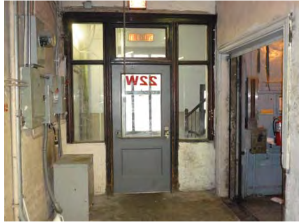
Image 78: Remaining storefront wall to west stair, 22 nd floor.
