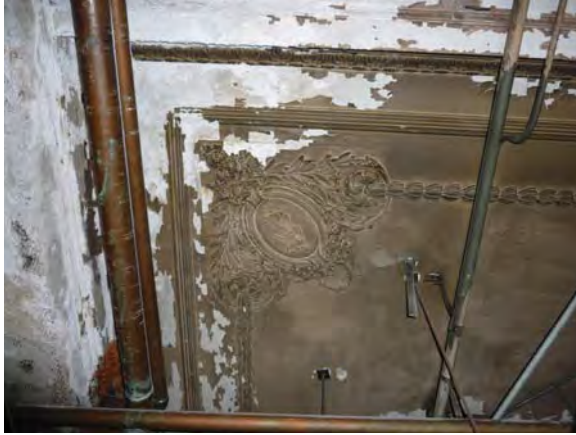
Image 51: 1 st basement, plasterwork on ceiling.
