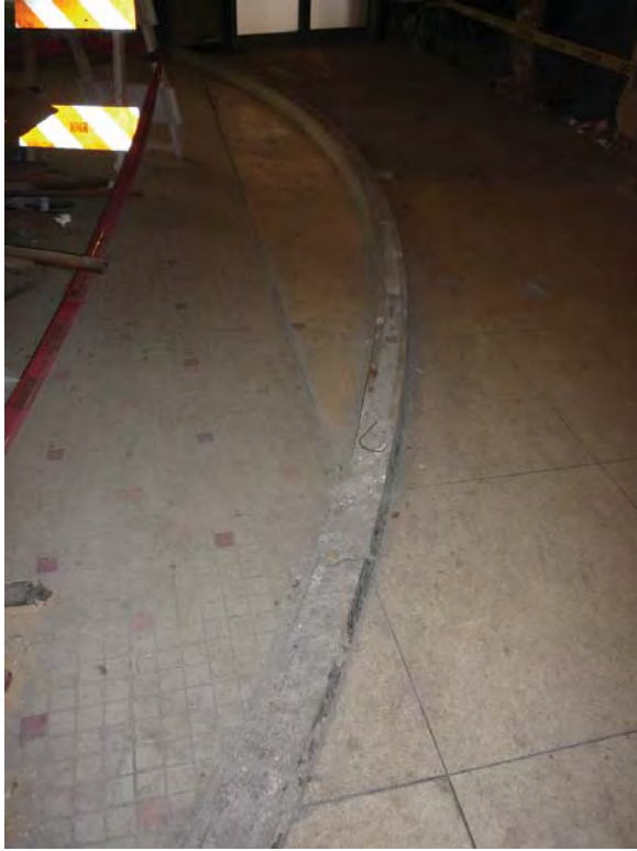
Image 67: Concrete frame for extinct curved glass wall.
