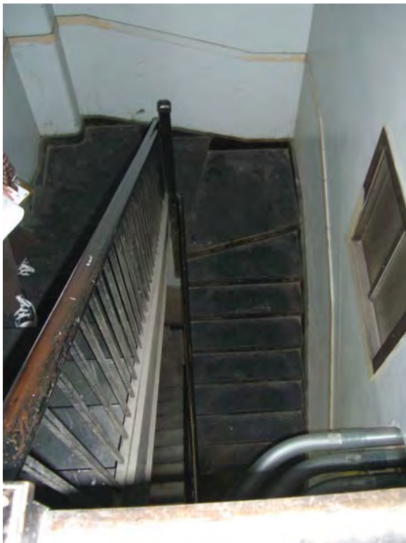
Image 65: West stair, slate treads between 22 nd floor and roof.
