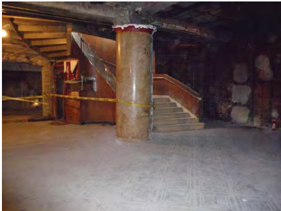
Image 37: First basement, view east to ornamental stair.
