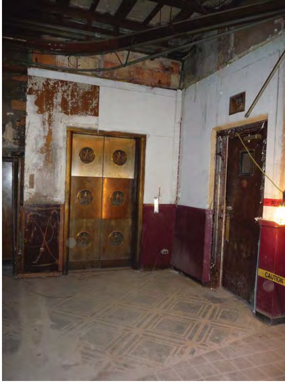
Image 39: First basement, elevator and main stair enclosures.
