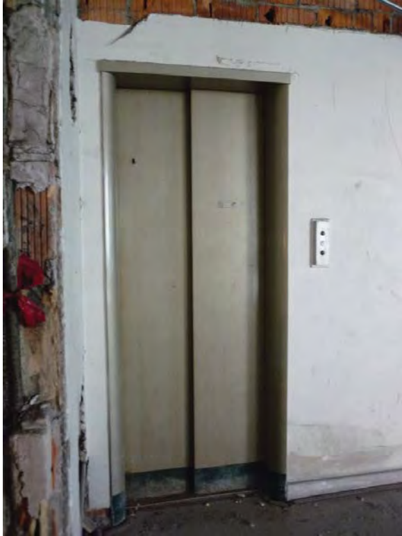
Image 51: West elevator enclosure.
