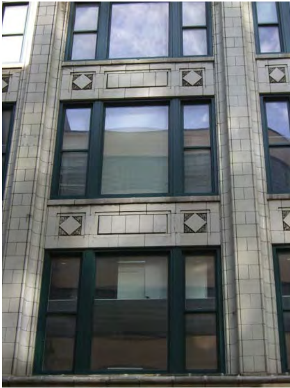
Image 29: Typical Chicago windows floors 2 through 4, east and south façades.
