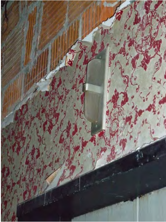
Image 47: Art Moderne hall call lantern above elevator doors, typical of floors 2 through 15.
