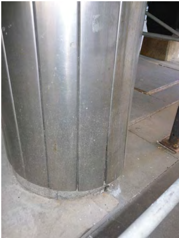
Image 61: Northeast exterior column and steel cladding.
