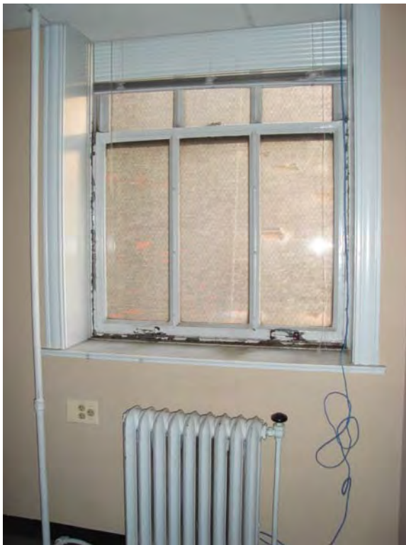
Image 93: North fire window, 7 th floor.
