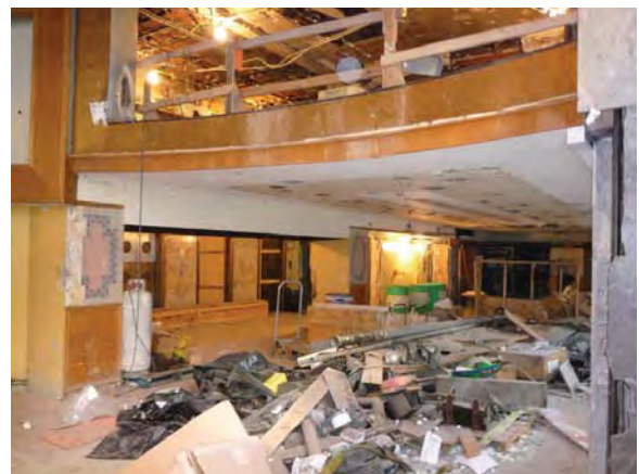
Image 34: First floor tenant space, view west.
