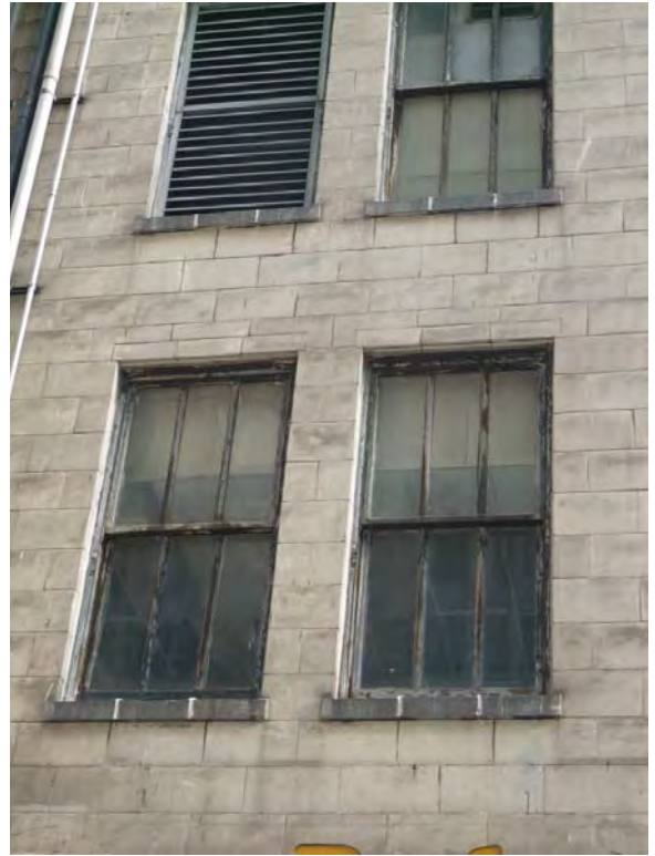
Image 30: Typical windows, west façade.
