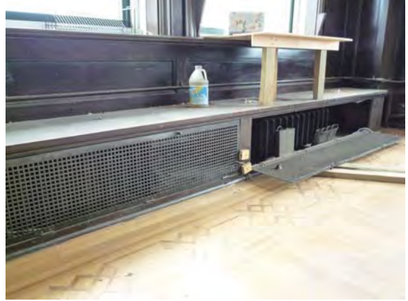
Image 76: 20 th floor, southeast office suite, remaining radiator enclosure.
