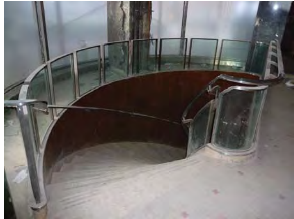
Image 36: Ornamental stair to first basement.
