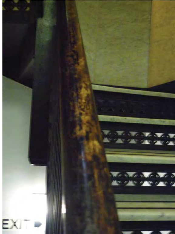
Image 112: Typical condition of railing finish, east stair.
