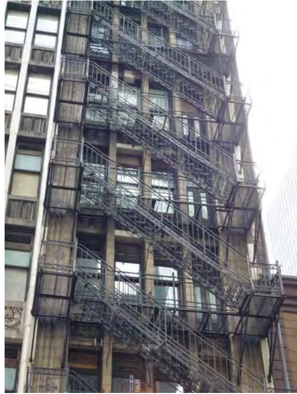
Image 28: Original fire escape, north façade.
