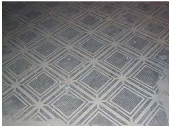
Image 38: First basement, mosaic tile floor.
