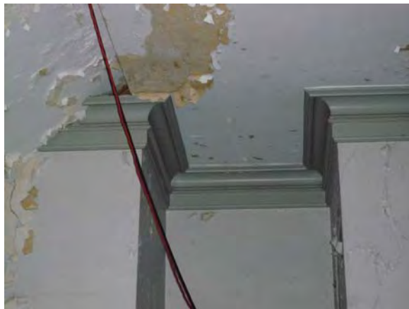
Image 53: Typical crown moulding above utility closet doors.
