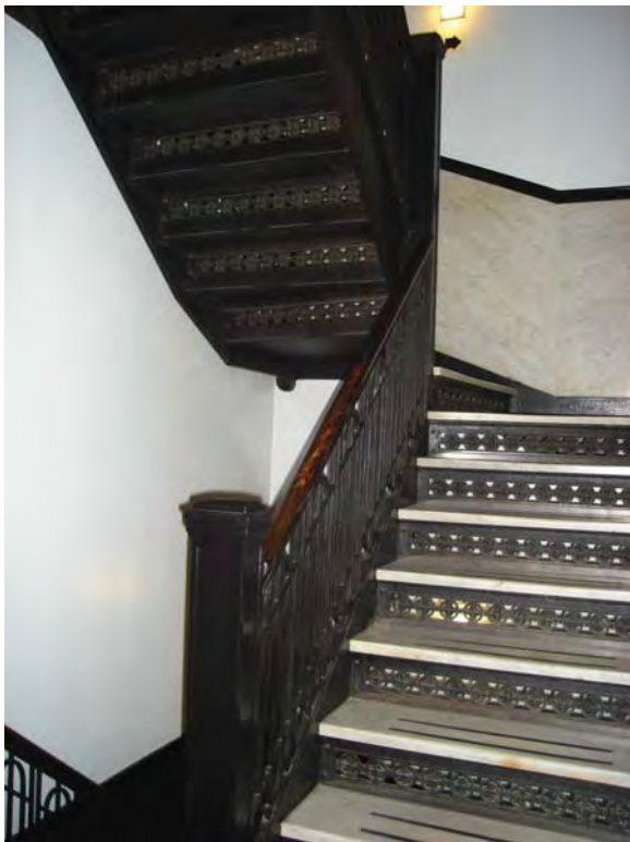
Image 61: East stair, marble treads and cast iron risers.
