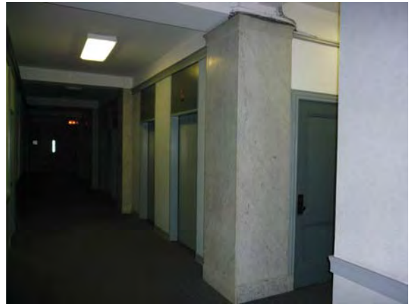
Image 84: Marble-clad columns in main corridor, typical of floors 2 through 21.
