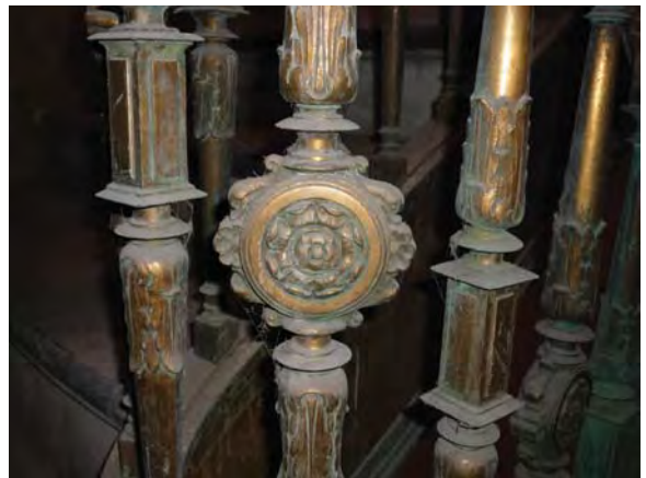
Image 42: Detail of bronze balustrade, main stair.
