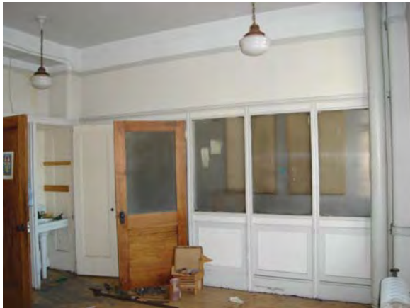
Image 73: 20 th floor, southeast office suite, partition wall.
