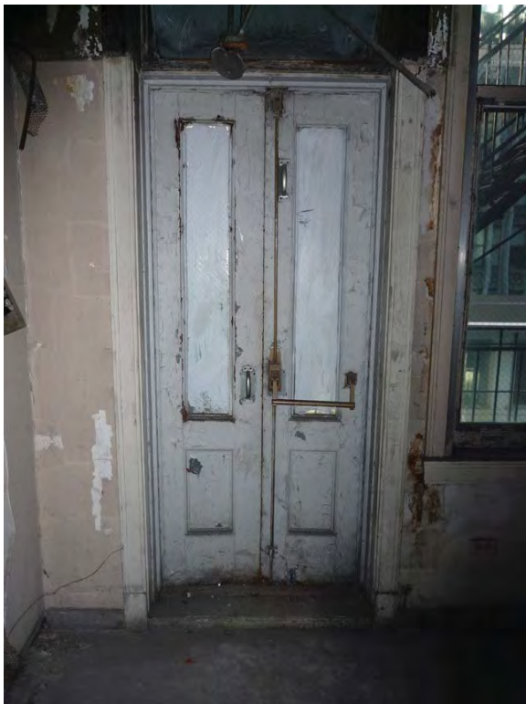
Image 57: 3 rd floor fire escape doors. Typical of floors 3 through 15.
