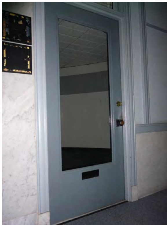
Image 82: Original door design, main corridor.
