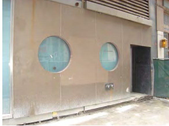
Image 76: Northwest entry, cladding over 1951 storefront.
