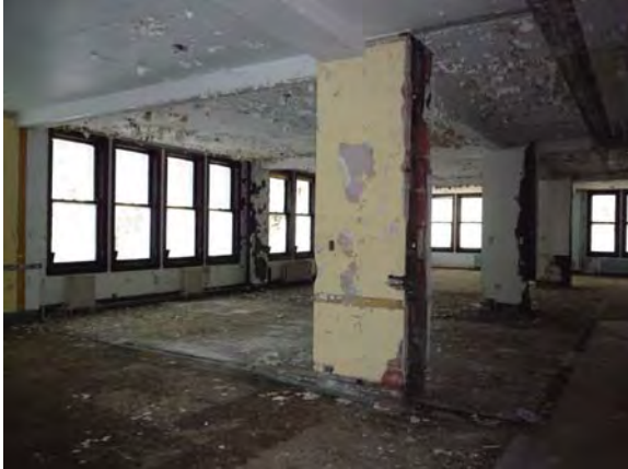
Image 81: 14 th floor tenant space. Typical condition of floors 2-15.
