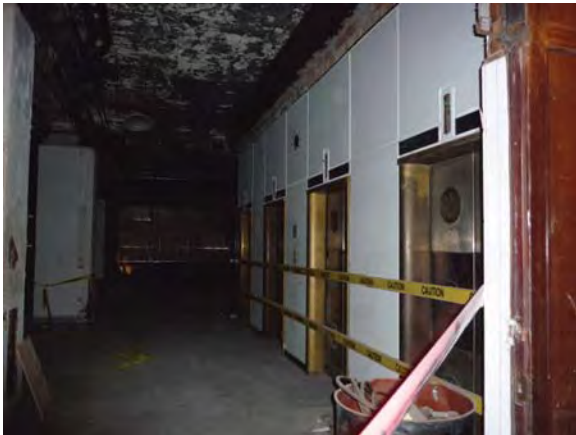
Image 73: Elevator doors, floor 2.
