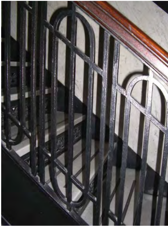
Image 59: East stair, cast iron balustrades and wood railing.
