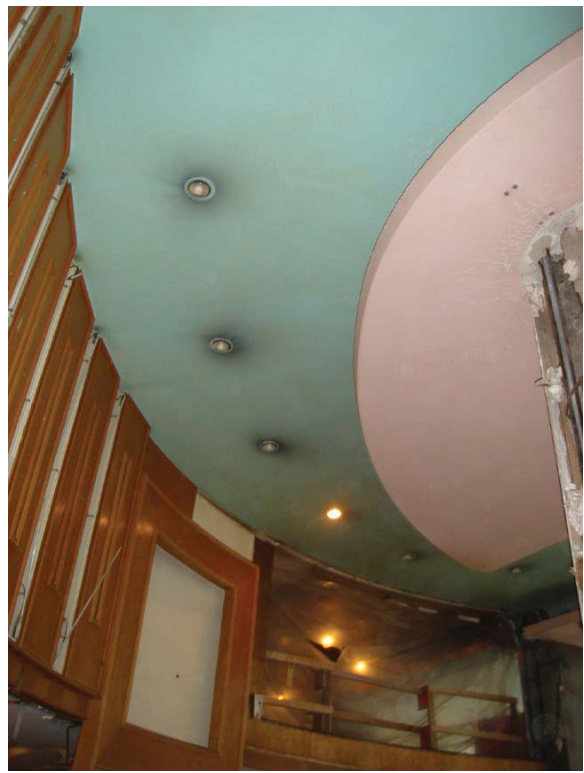
Image 78: First floor tenant space; 1951 lighting and ceiling.
