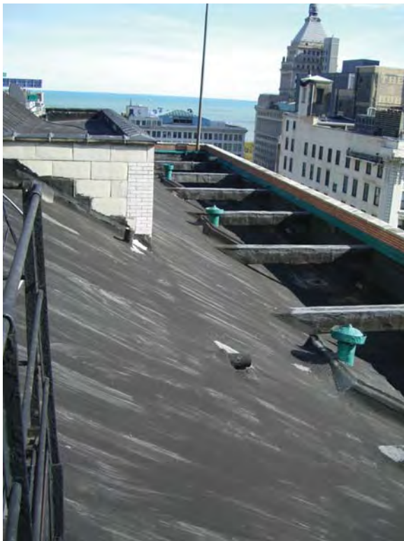
Image 101: Rooftop, view east.
