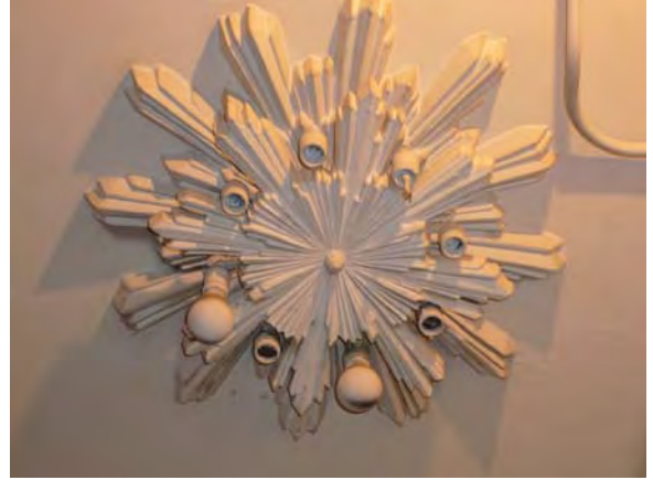
Image 52: 1 st basement, ceiling light fixture.
