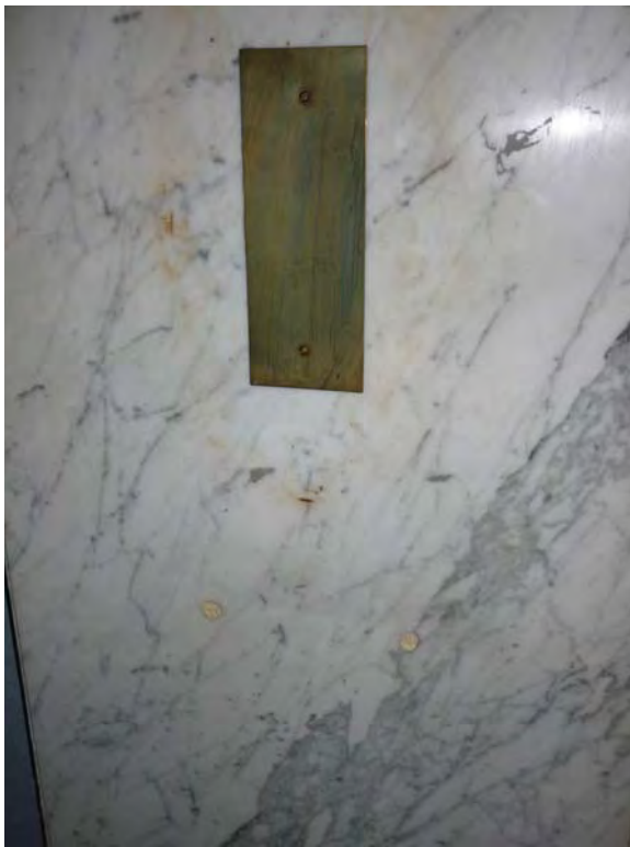
Image 105: Typical marble condition, elevator lobby, floors 2 through 21.
