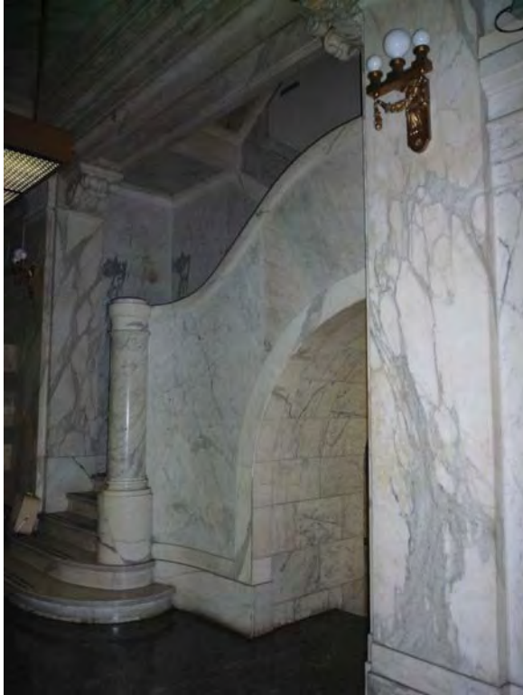
Image 55: East stair, first floor.
