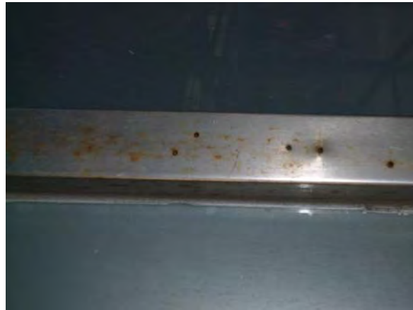
Image 60: Steel storefront frame, east façade.
