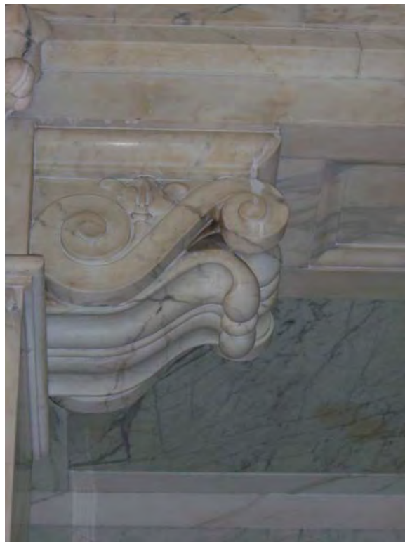
Image 58: Decorative bracket, east stair, first floor.
