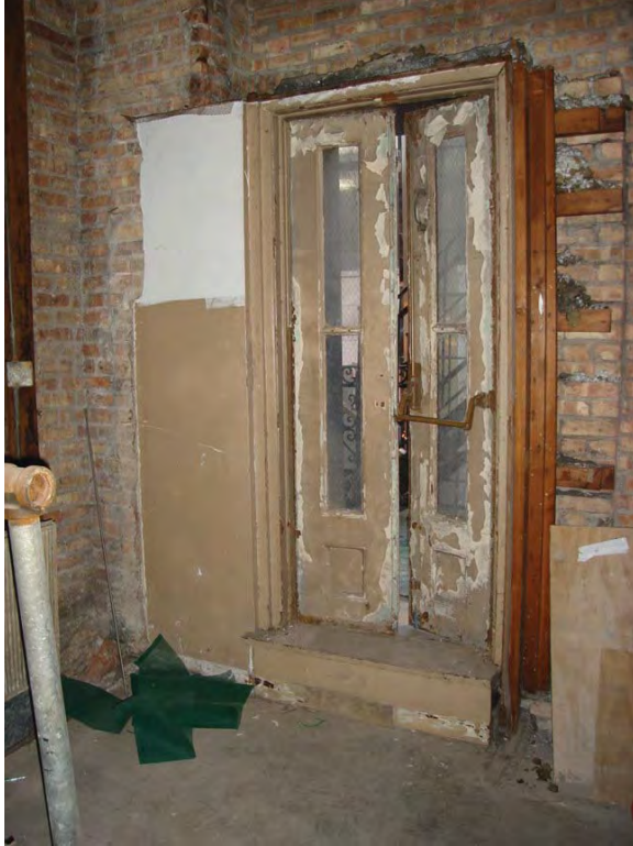
Image 55: 2 nd floor fire escape doors.
