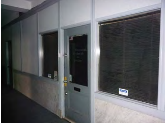
Image 79: Remaining storefront wall, main corridor 13 th floor.
