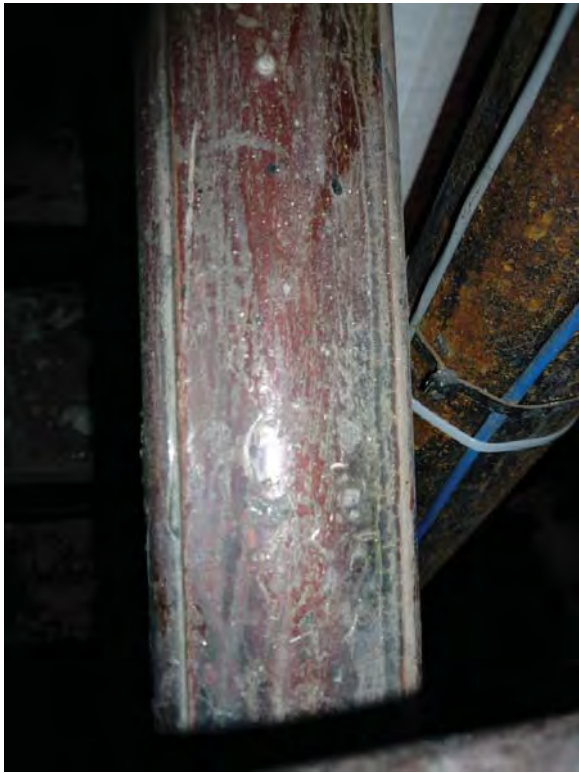
Image 69: Typical railing condition, main stair, mezzanine and above.
