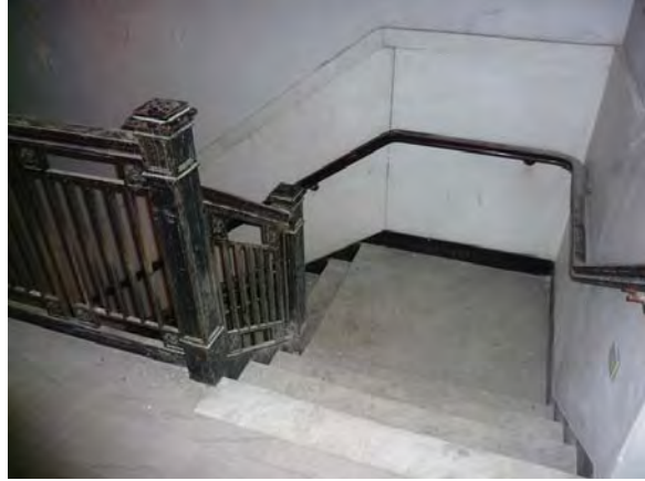
Image 44: Main stair, typical floors 2 and above.
