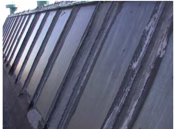
Image 102: Rooftop skylights, view west.
