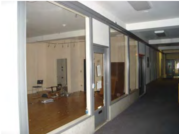
Image 77: Remaining storefront partition wall, main corridor 4 th floor.
