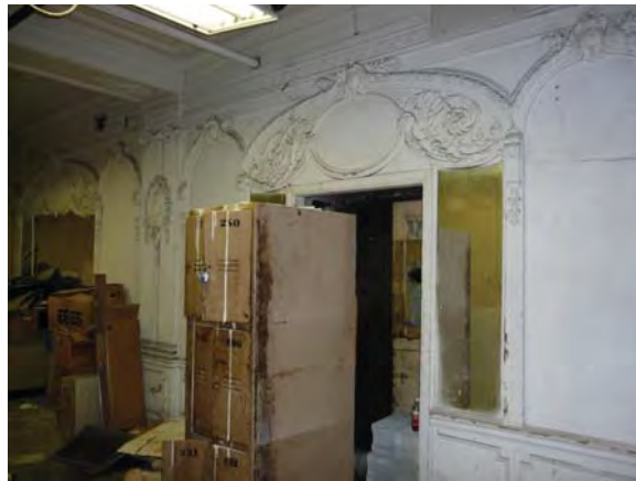
Image 48: 1 st basement, decorative plasterwork.
