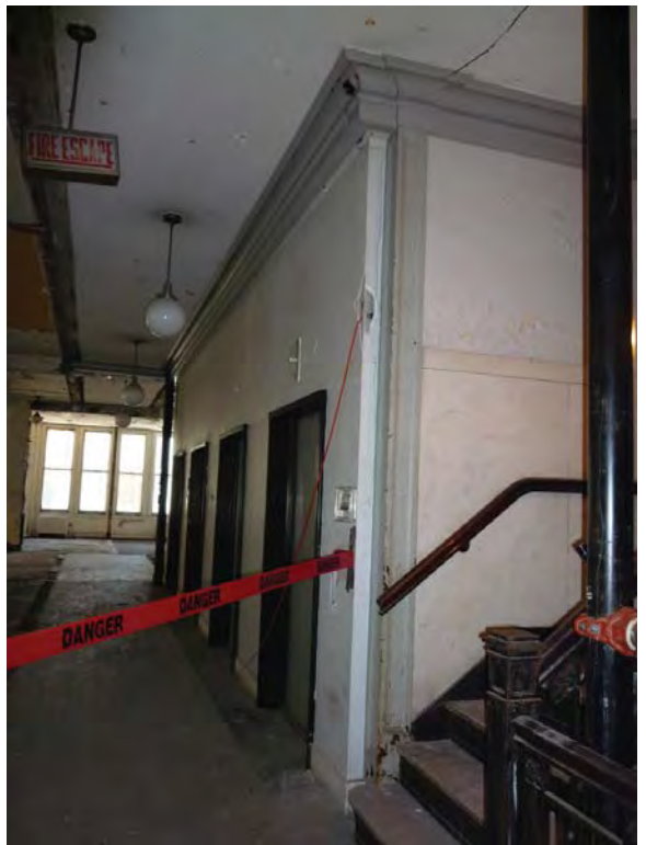
Image 74: Elevator enclosure and doors, typical of floors 2 and above.
