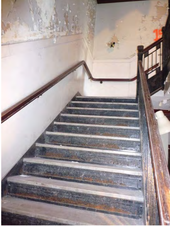
Image 43: Main stair, typical floors 2 and above.
