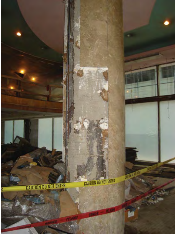
Image 79: Cylindrical column, first floor tenant space.
