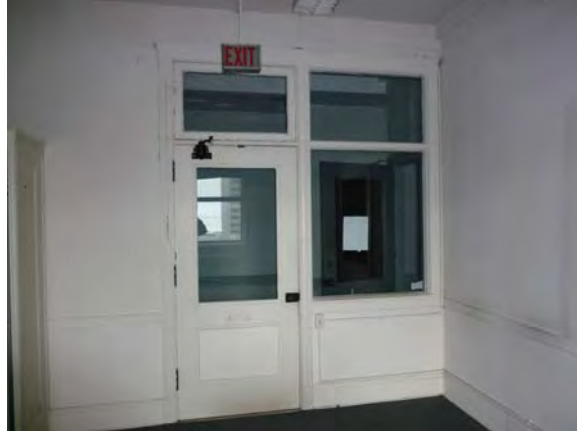
Image 80: Remaining partition wall, east office, 14 th floor.
