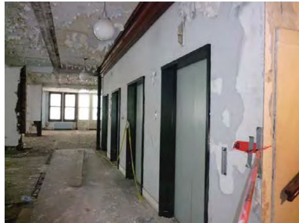
Image 52: Typical elevator enclosure, floors 2 through 15.
