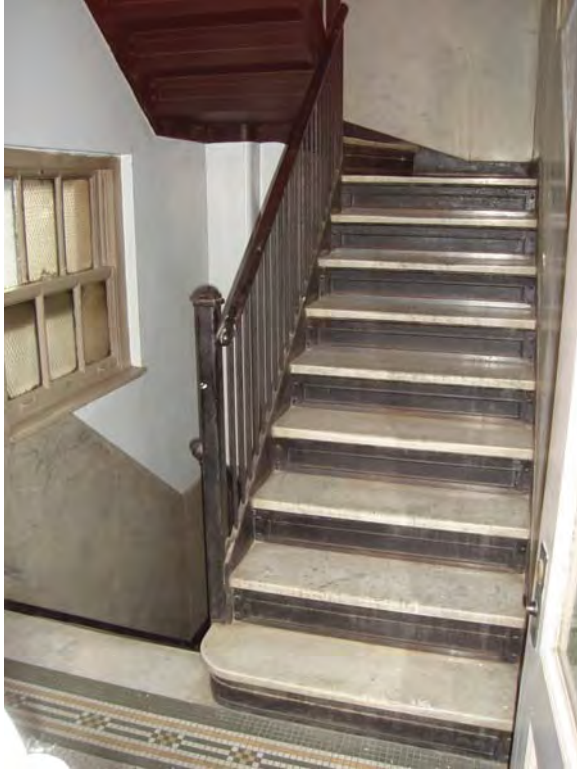
Image 63: West stair, cast iron structure and marble treads.
