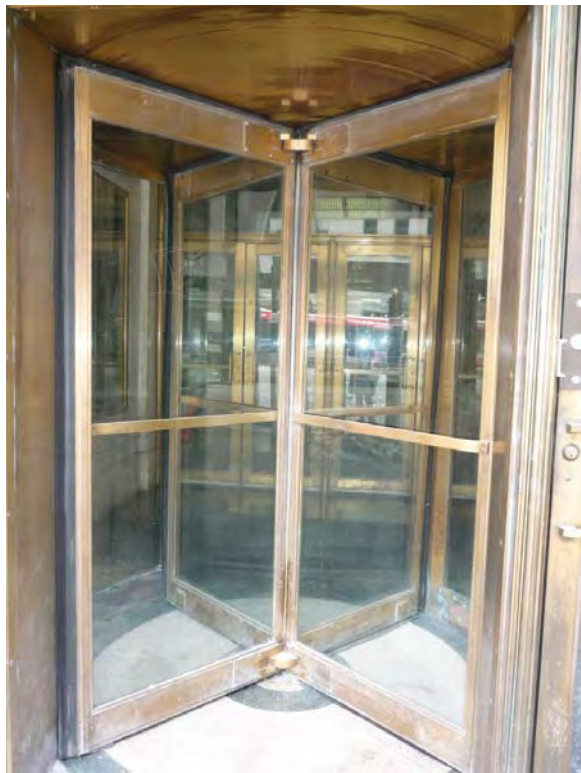
Image 33: Existing revolving door.
