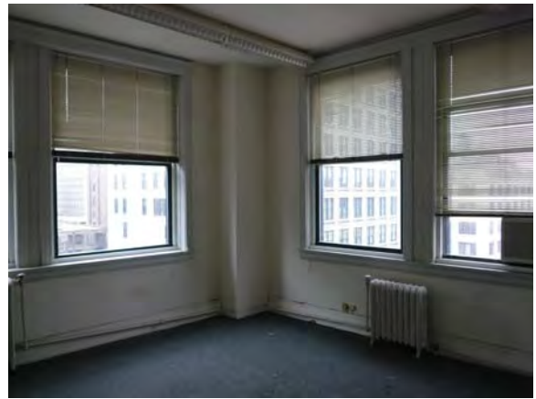
Image 92: East and south windows, 13 th floor. Typical of floors 5 through 21.
