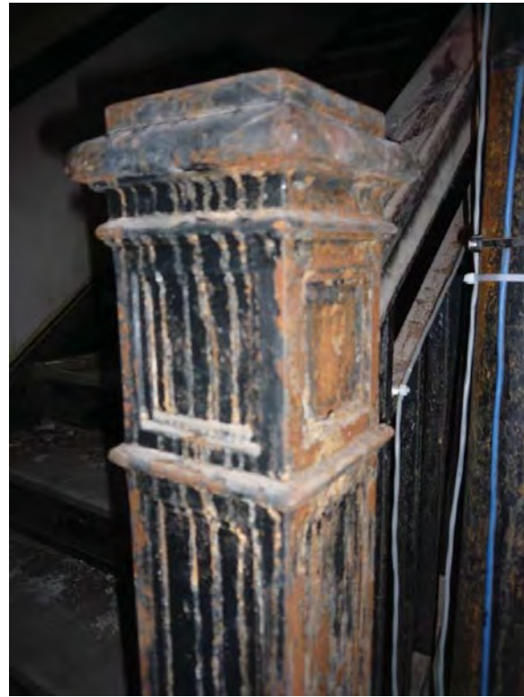
Image 70: Typical newel post condition, main stair, mezzanine and above.
