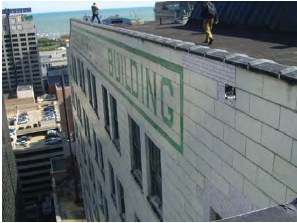
Image 23: North façade signage.
