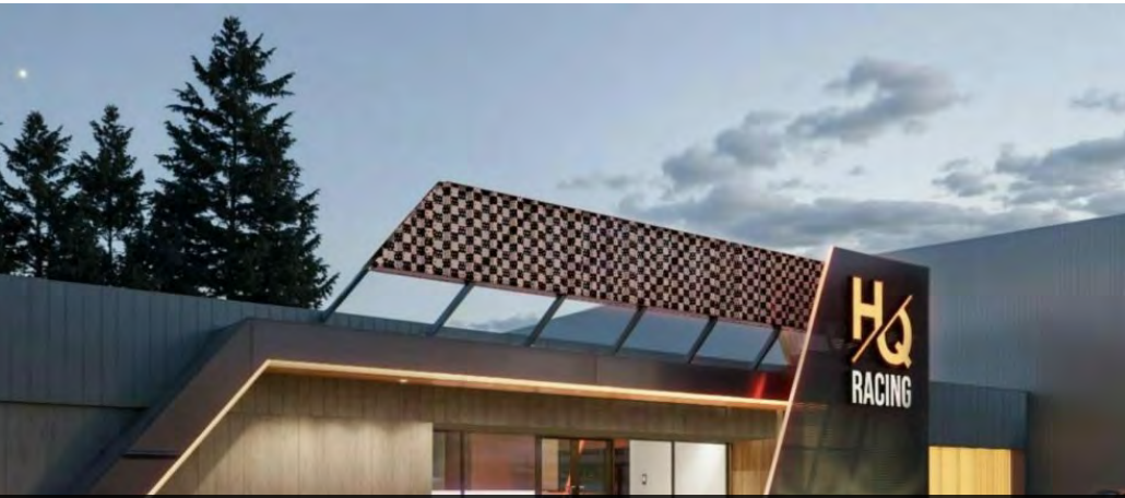
The new race track in Peekskill, NY, is a large-scale indoor/outdoor electric go-kart track called HQ Racing, which is scheduled to open in Fall 2025. It will feature a multi-level track, designed to be the largest of its kind in the United States, with options for various skill levels and accessible karts for people with disabilities. The project is being developed in the former HQ Auto Vault building at 7 John Walsh Boulevard.
