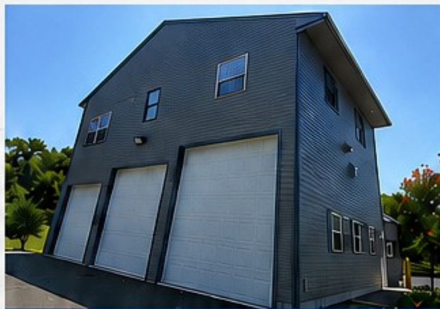
SIDE VIEW – 3 GARAGE DOORS
